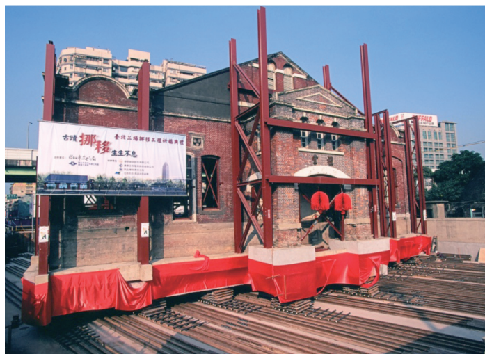
Removal of historic relics at the Songshan Line's Beimen Station
