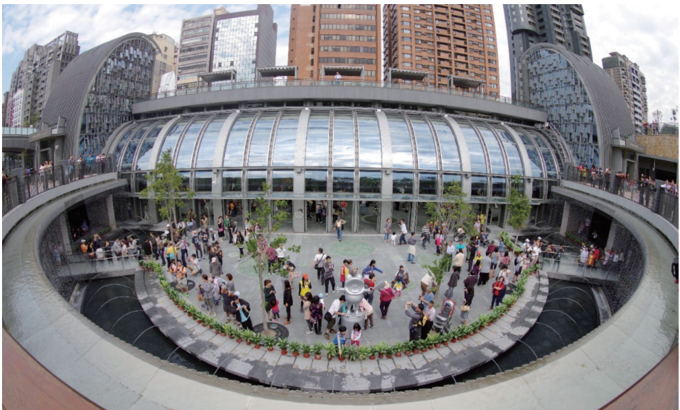
Daan Park Station
