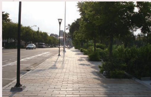
Sidewalk on the north of Jiuquan Street after illumination improvements
