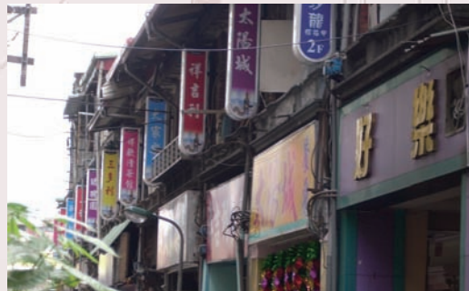
Lane 212, Section 1, Xiyuan Road of Wanhua District after renovation
