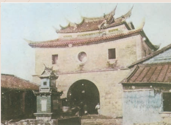
●The West Gate being torn down
