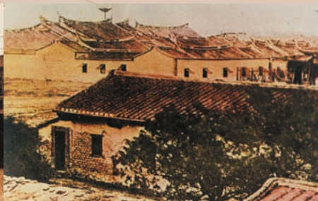
● The Governor's Building of the Official Governor of Taiwan commissioned by the Qing Dynasty
