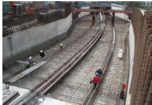
CL700B區段標之CL804標蘆洲站出土段軌道版鋼筋綁紮
