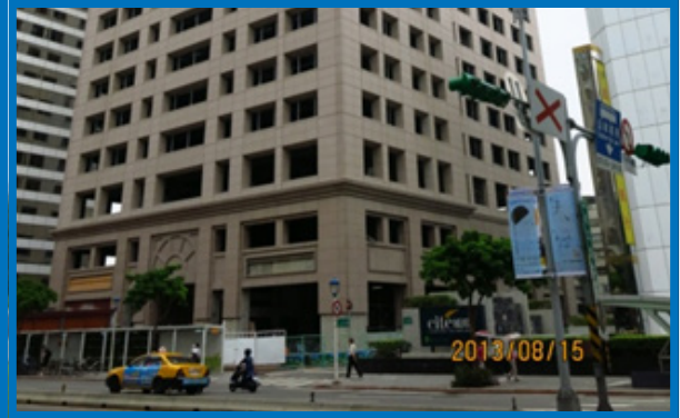
Xingtian Temple Station (M8) JD project under construction
