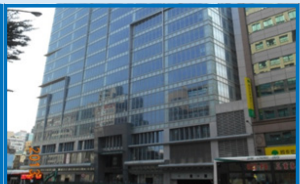
Nanjing Fuxing Station (M4) JD project under construction
