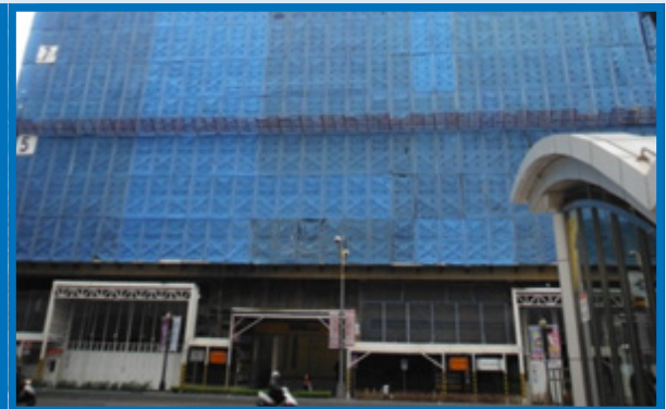
Cailiao Station (M4) JD project under construction
