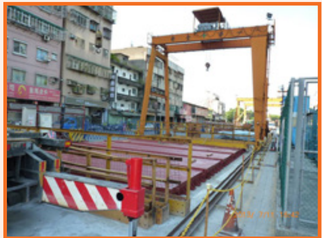
Assemblage of flood prevention cover plates at track input port
