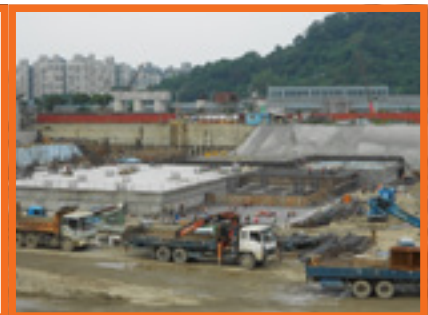
Construction of foundation decks at the South Depot fan-shaped track area
