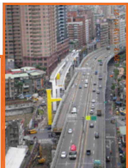
A viaduct beside ramps leading to Yixia Bridge, Zhonghe on Provincial Highway No. 64
