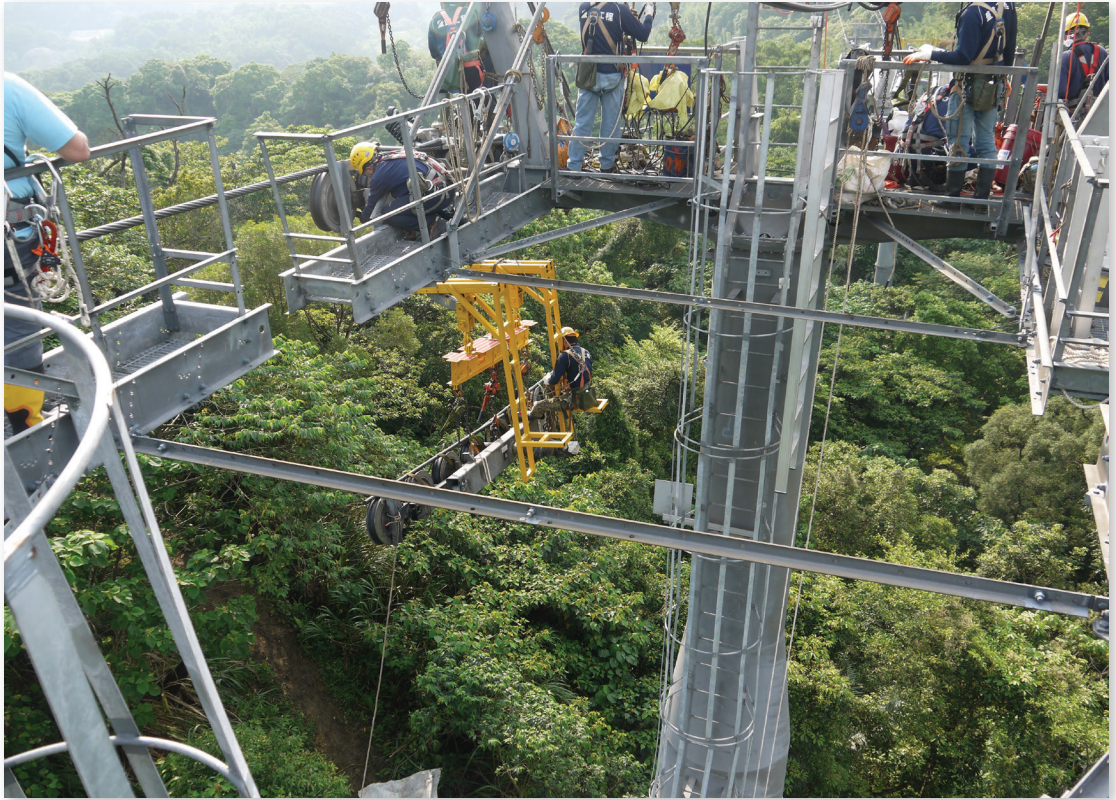
The first Overhaul of important equipment began on May 2, 2012
