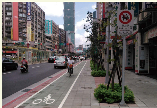
The MRT Xinyi Line project to restore streets to pre-construction condition including new bike lanes
