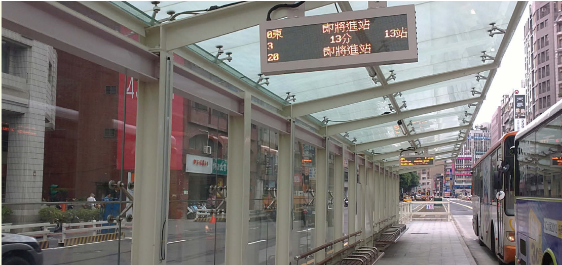
Installing intelligent bus stops along the MRT Xinyi Line
