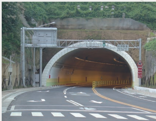
Kanghu Road opened to vehicular traffic
