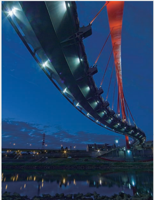
Night views of the pedestrian overpasses across Xinming Road in Neihu and Raohe Street in Songshan
