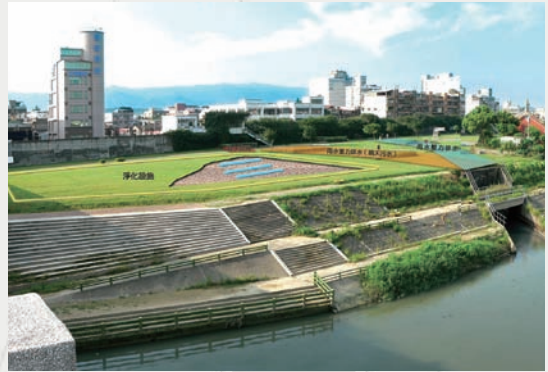
Site of the Chengmei Rainwater Pumping Station
