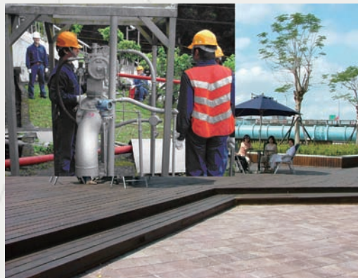
Natural gas pipeline security repair drill
