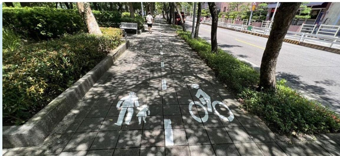
Pedestrian-vehicle separation lines have been added along the east side of Songde Park, ensuring cyclists stay close to the roadside and pedestrians walk on the building side without disturbing one another.
