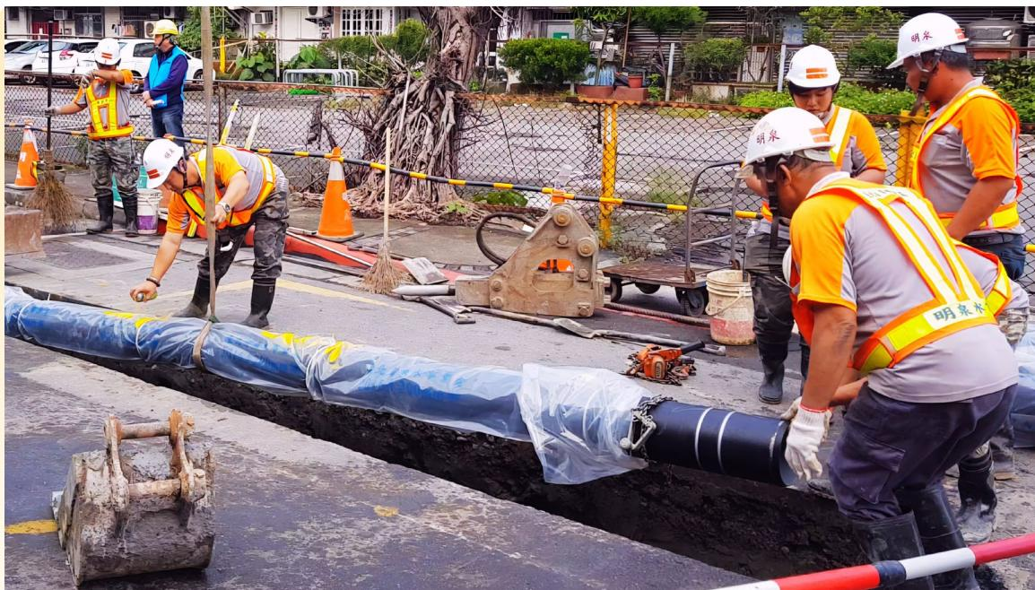
In pipeline replacement optimization projects, high-quality pipe materials are used to improve water quality.
