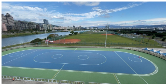
為 113 年中運整修迎風競速滑冰場 Yingfeng Roller Skating Rink for the 2024 National High School Games
