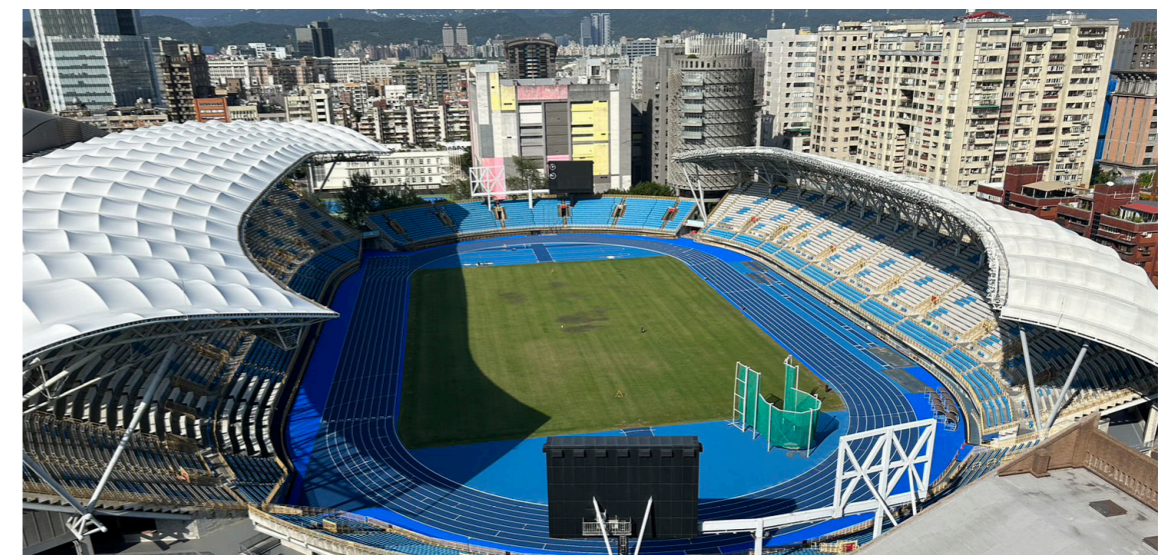
臺北田徑場跑道翻新 Taipei Municipal Stadium track resurfacing
