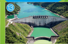
13 Feitsui Dam Feitsui dam is a "3-centered double curvature variable thickness concrete arch dam", and its beautiful geometry is unique in the country.
