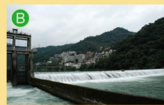
B Tsungling Dam retains the water from Xindian Creek. The water is diverted to Tsungking Power Plant for power generation and part of the water flows to Chihitan reservoir for tap water use.
