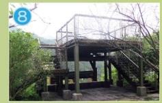
8 Scenic Lookout Here is the best spot to enjoy the magnificent view of the downstream valley. You can see the whole picture of the dam and its facilities. If you bring a binocular, you may also see Crested Serpent Eagles hovering over the sky. Good Luck!
