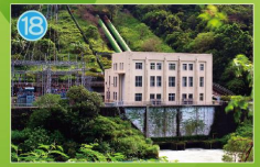
18 Guishan Hydropower Plant Guishan Hydropower Plant, built in 1939 and owned by Taiwan Power Company, is a run-of-river power plant with an installed capacity of 15,000KW. It is the administration and remote control center of all the hydropower plants of Xindian Creek System.
