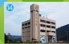
14 Operations Building The secondary operations center in the building is in charge of controlling and monitoring the operations of releasing facilities; it also manages the emergency situations.
