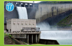
17 Feitsui Hydropower Plant To fully utilize the hydropower, Feitsui Power Plant was established in the downstream of Feitsui Dam. With the total capacity of 70MW, the average annual power generation is about 220 GWH, which equals to a total reduction of 116,000 tons of CO2e per year.
