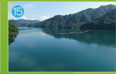
15 Trash Boom The main function of the trash boom is intercepting driftwoods and debris in the reservoir, avoiding the impact to the dam and hydraulic machinery facilities, ensuring the dam and reservoir operation safe.
