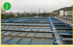
I Changhsing water purification plant yields more than 543,000 tons of tap water daily.
