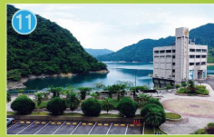
11 Dam Area Park With the assistance of Hsi Liu Environmental Greening Foundation, the park is designed with colorful ground, streamline flower platform, flowers and trees.
