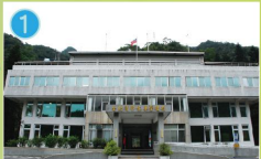
1 Administration Building The staff in the administration building are in charge of dam safety, reservoir operation and watershed management.
