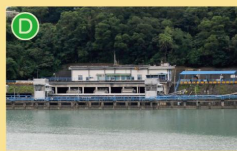
D After Chihitan intake collects water from Xindian Creek, the water is then distributed to Chihitan purification plant via the water tunnel.
