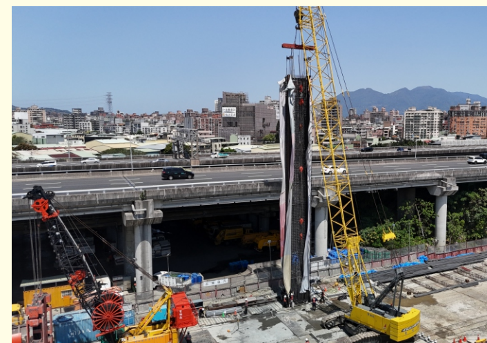
▲ 北環段Y19B站連續壁工程施工 North Section Station Y19B Diaphragm Wall Construction
