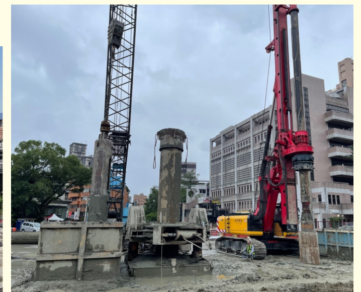
▲ 南環段Y1A站密排樁工程施工 South Section Station Y1A Dense Pile Construction
