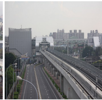
Construction status of Station G16 and entrances/exits along Jianguo Road
