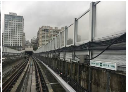
Sound barrier for daylight section
