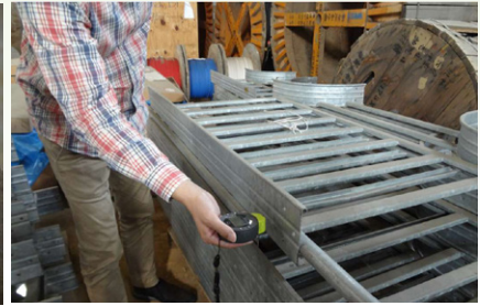
Inspection of signal cable troughs inspection
