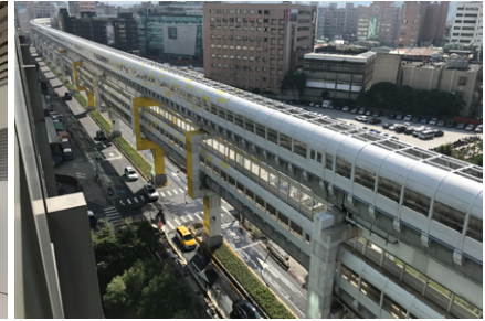
Completion of the noise barriers on the viaduct along Bannan Road and planting in the median island
