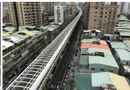
Current completed status of noise barriers along Banxin Road
