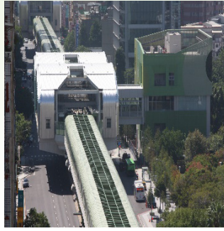
Current construction of Station G10a and entrances/exits along Wenxin Road
