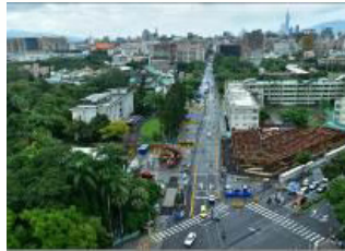
Bird's eye view of station excavation on the south side along Nanhai Road and ground level structure construction at Mandarin Experimental Elementary School integrated building site
