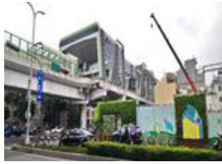
Construction of Station G8 from Ningxia Road to Henan Road
