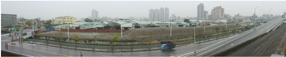
Fig. 2: The ballast stacking area at the tail track section of Taipei MRT Luzhou Linear Park
