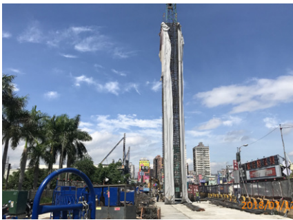
Diaphragm wall rebar cage hoisting of cut-and-cover tunnel section at Sec 3, Jingcheng Road
