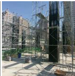
Station G6: structural engineering of land development building--3F structural formwork rebar-binding operation
