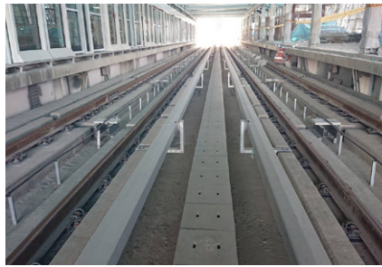
Banqiao Station construction of station main structure and track
