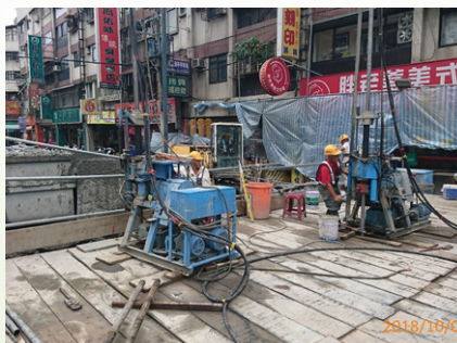
Middle piles construction at Station LG08
