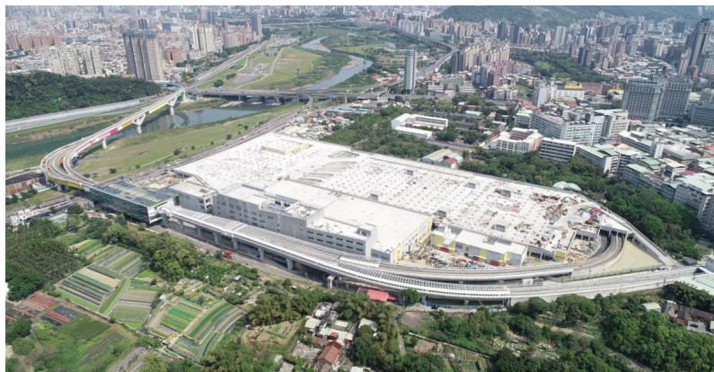
Current Status of South Depot
