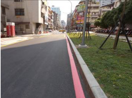
Road restoration on Minquan Road
