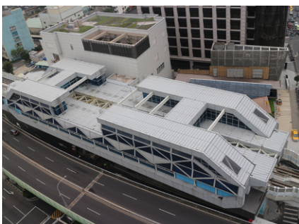
Finishing works of Touqianzhuang Station
