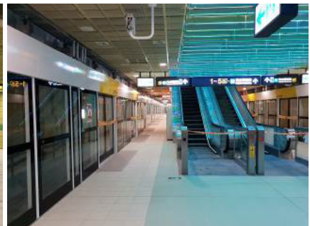
The completion status of the platform
