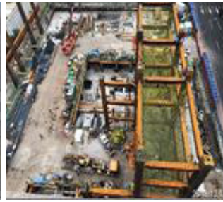
Station G09-1: Lifting of steel structure
