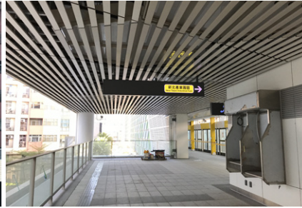
Ceiling and signals at the connecting zone of Zhonghe Station
