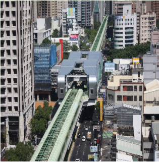
Current construction of Station G10 and entrances/exits along Wenxin Road
