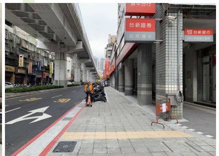
Sidewalk widening in the non-collinear section along Jingping Road
