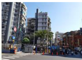
Dewatering well construction
