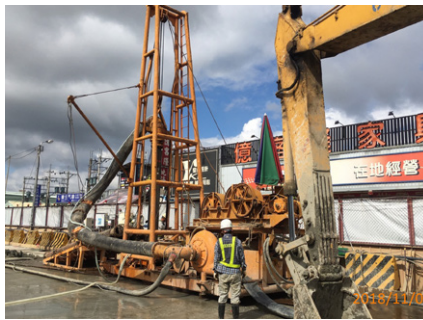
Middle piles construction of the cut-and-cover tunnel section at Sec. 3, Jingcheng Road
