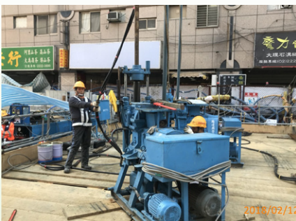
Stratum improvement of the launching well at the shield tunnel of Station LG08
