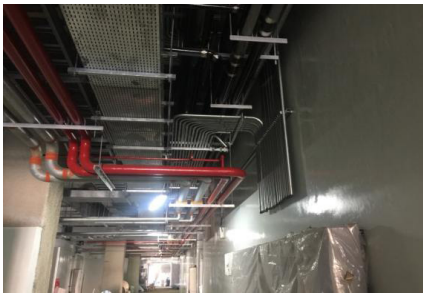
Xinpu Minsheng Station construction of electric system and chilling water pipelines
