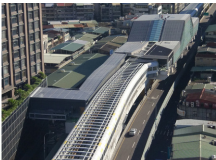
Elevated Jingan Station
