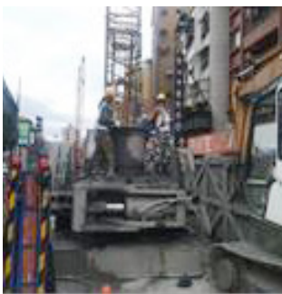
Construction of full sleeve construction of middle columns in the central shelter line
