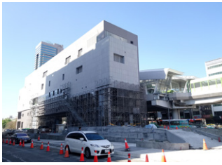
Construction of Station G7 from Zhongqing Road to Xiayi Road
