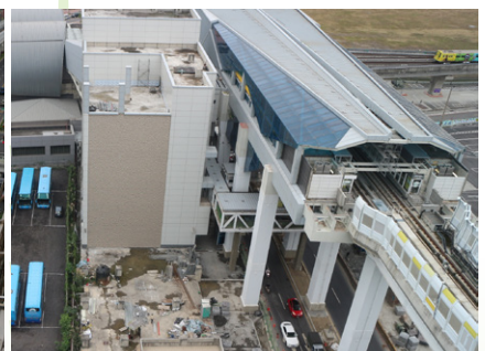
Construction of New Taipei Industrial Park Station and land development building
