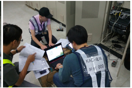
Optic fiber transmission system acceptance tes
