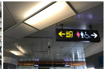
Ceiling and signals at the concourse of Banxin Station
