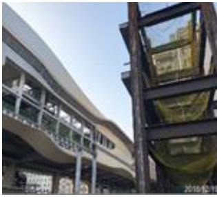
Station G09-1: installation of steel columns/beams at passage handover zone
