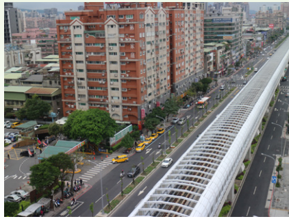
Construction of noise barrier between the elevated Touqianzhuang Station and the elevated section of Xingfu Station
