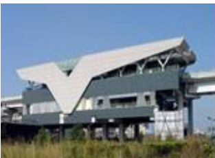
Construction of Station G3 from Jiushe Lane to Hanxi West Road
