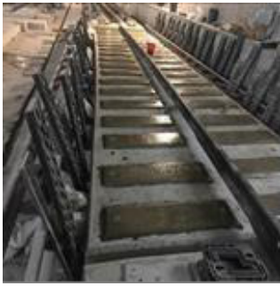
Construction of the turnout base in the mountain tunnel
