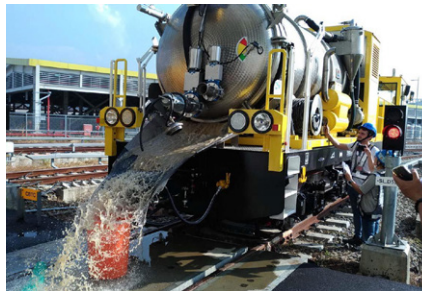
Mud-sucking truck site test
