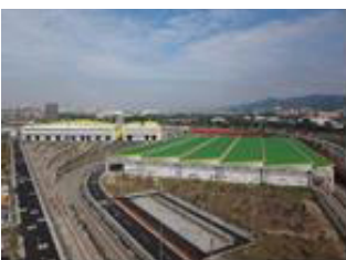
Primary maintenance plant /track maintenance plant/ north stabling yard
