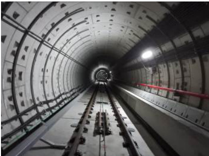
Completion of shield tunnel
