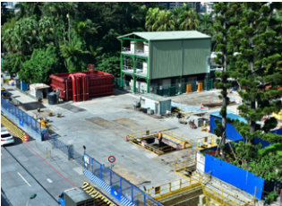
Construction of Jingmei layer dewatering operation at station site
