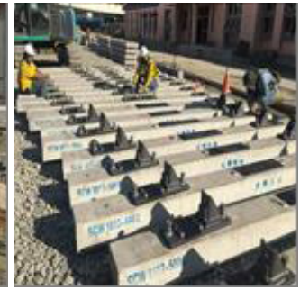
Positioning of the turnout bed in the sect area turnout
