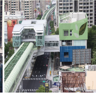
Current construction of Station G12 and entrances/exits along Wenxin Road
