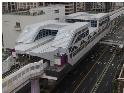
Finishing works of Xingfu Station
