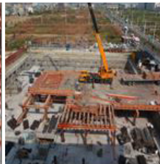
Construction of stage 1 excavation support and removing of decking
