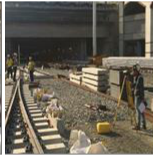
Survey operation of the ballast pavement in the sect area
