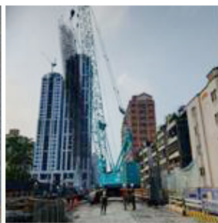
Construction of diaphragm walls at the north side of Station LG05 (hoist rebar cages)
