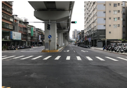
Elevated section construction of Banxin Road restoration
