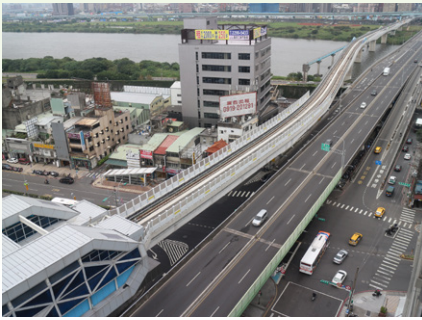
Construction of noise barrier between the elevated stations across the Dahan River to Touqianzhuang Station
