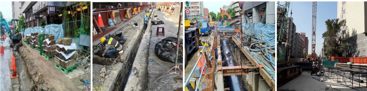
Relic structure of formal gutter made in the Japan-controlled era
