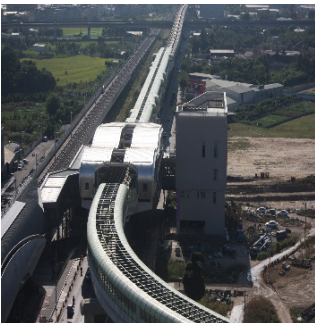
Construction status of Station G13 and entrances/exits along Jianguo Road
