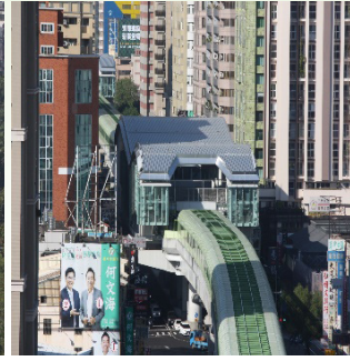
Current construction of Station G11 along Wenxin Road
