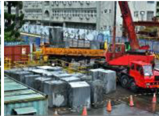
Station entrance A diaphragm wall chain-cutting operation
