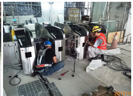
Installation of automatic fare gates
