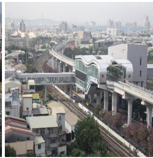
Construction status of Station G15 and entrances/exits along Jianguo Road
