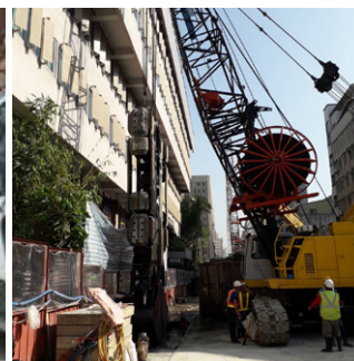
Construction of diaphragm wall
