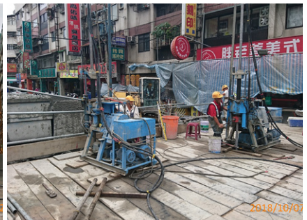
Stratum improvement of the arriving well at the shield tunnel of Liancheng Road
