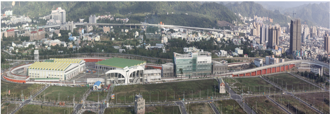
Bird's-eye view of the entire construction area
