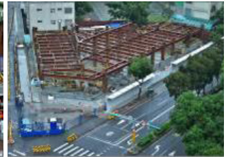
Ground level structure construction at Mandarin Experimental Elementary School integrated building
