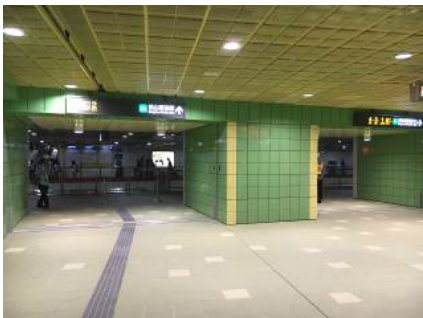
Connecting tunnel to Dapinglin Station on the Xindian line
