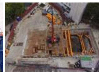
Construction of retaining support and decking for the working well at Yucheng Park
