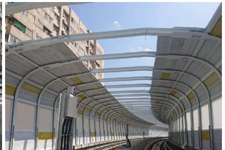
Construction of noise barriers on viaduct section
