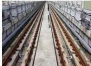
Completion of track and conductor rails
