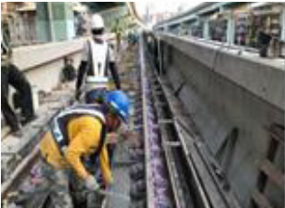
Concrete plinths placement
