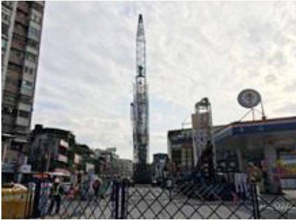
Hoisting and erection of rebar cages for the diaphragm walls
