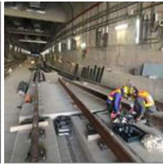
Construction of the ballast-free bed base in the mountain tunnel
