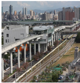
Construction status of Station G14 and entrances/exits along Jianguo Road
