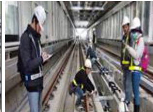
Post-installation inspection of conductor rails
