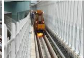
Initial rails grinding
