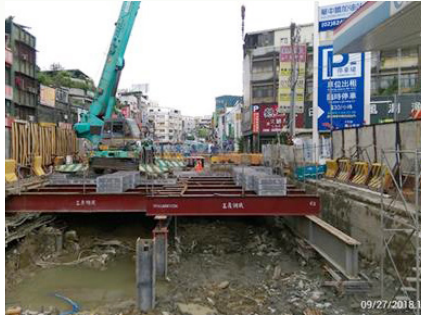
Installation of decking beams
