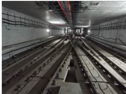
Completion of cut-and-cover tunnel
