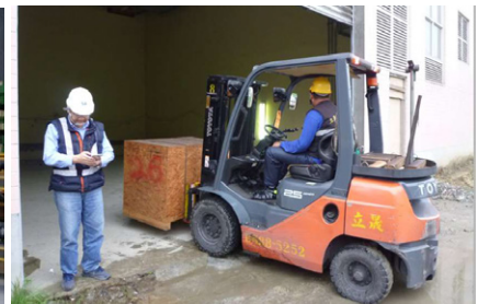
Arrived depot equipment is delivered to site
