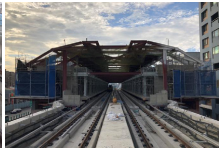
Xinpu Minsheng Station construction of station main structure
