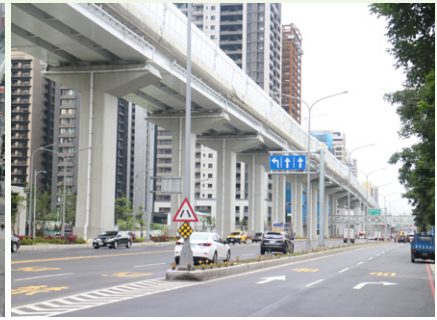
Noise Barriers between Xingfu Station and New Taipei City Industrial Park Station, and beneath the elevated station, the median island between the section
