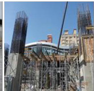
Station G11: structural engineering of land development building--3F structural formwork rebar-binding operation
