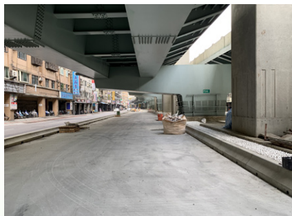
Motorcycle area inside the median island in the collinear section along Jingping Road
