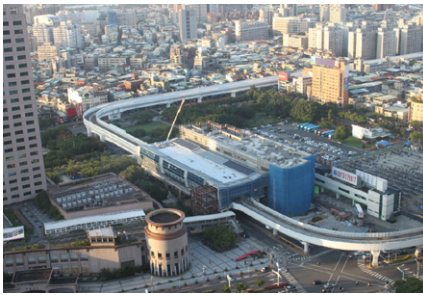
Banqiao Station construction of station main structure and land development building
