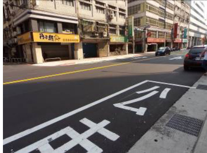
Road surface restoration on Minquan Road
