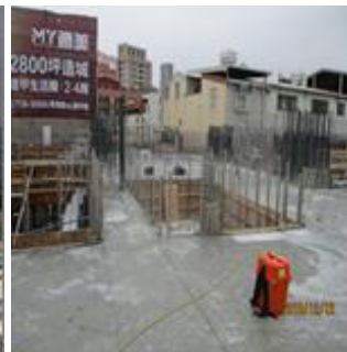
Station G8a: structural engineering of land development building--2F floor curing operation
