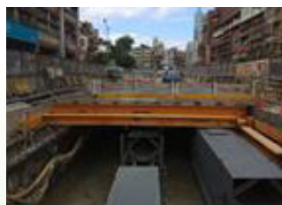
Construction of Station R03 temporary drainage steel aqueduct
