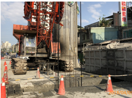
Excavation works for the diaphragm walls at Station LG07
