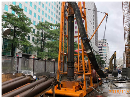
Erection of middle piles on the pocket track along Liancheng Road
