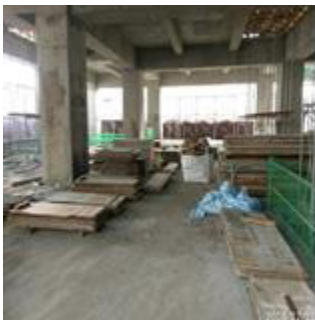
Station G5: structural engineering of land development building--2F structure formwork demoulding
