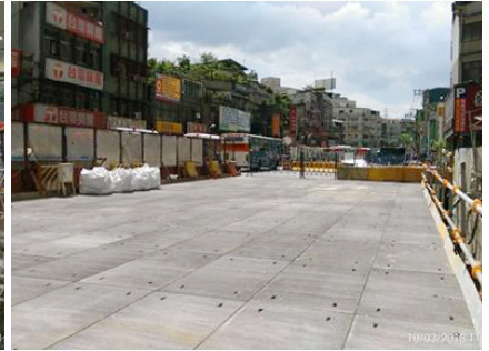
Setting up of decking
