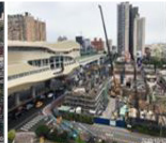
Station G09-2: 1F formwork assembly and rebar installation at 1F
