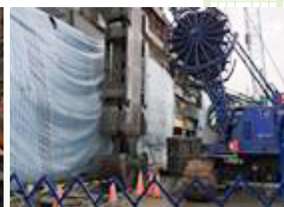
Construction of diaphragm wall south of Station R03
