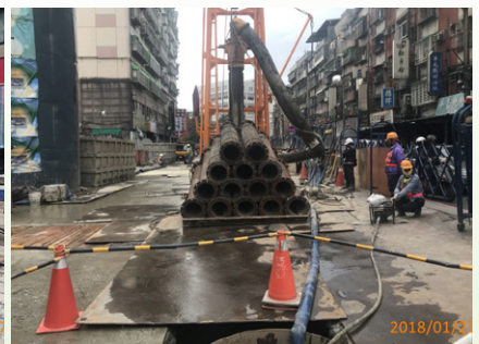
Decking construction at Station LG08
