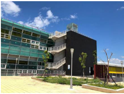
Shisizhang Station and landscaping platform
