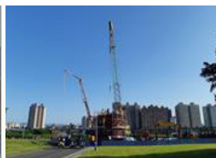
CP3 caisson construction
