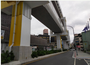
Road surface restoration on Zhongshan Rd. Sec. 2, Zhonghe
