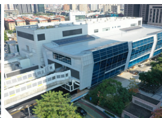
Banqiao Station and land development building (Circular line)
