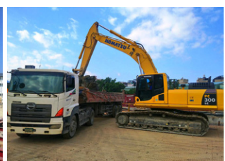
Excavation work at Station LG08A (Area 3)
