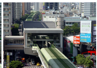
Construction of Station G6 from Chongde Road to Hebei Road
