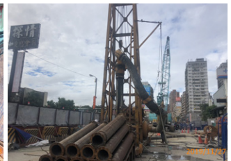
Boring for piles in the cut-and-cover tunnel on Jincheng Rd. Sec. 3
