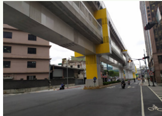
Surface restoration on Bannan Rd., Zhonghe
