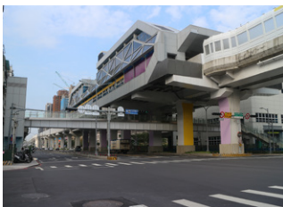
Xingfu Station (Y18) and Xingfu overpass
