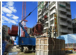
Station LG03 north diaphragm wall construction
