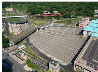
Aerial shot of track laying completed at Xingzhuang Depot
