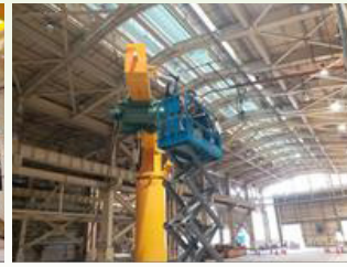
Jib crane installation at Xinzhuang Depot
