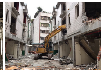
Demolition of buildings around Exit B
