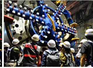
Shield tunnel machine assembly
