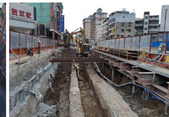
West side shallow excavation
