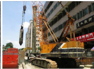
Station LG01 middle column work
