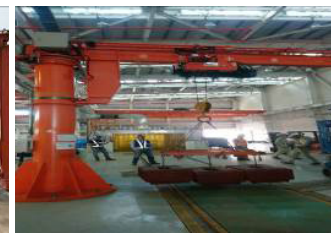
Depot equipment, jib crane on-site test
