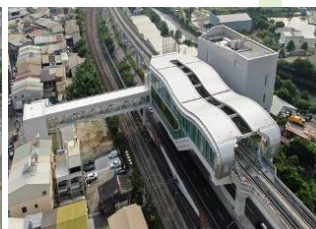
Construction status of Station G15 with entrances/exits along Jianguo Road
