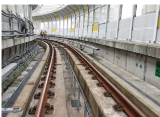
Line track and conductor rails completion
