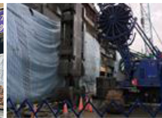
Construction of diaphragm wall north of Station R03
