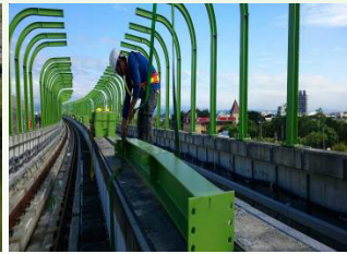
Jianguo Rd. sound barrier works
