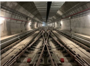
The turnout installation in the mountain tunnel is completed
