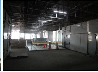
Station G3 Concourse
