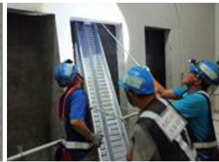
Communication system - cable trough work
