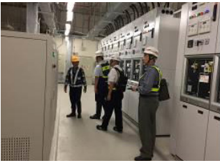
PWR, station equipment and construction examination
