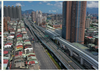
Elevated section of Xinpu Minsheng Station
