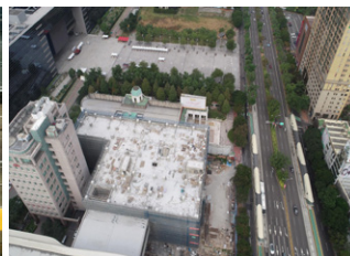
Station G09-1: current structure
