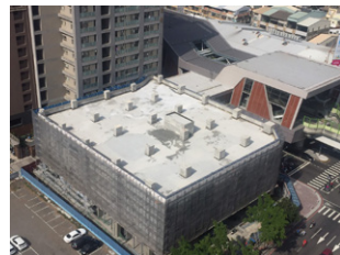
Station G6: Exits/ Entrances construction at Wenxin Rd. and Chongde Rd. intersection
