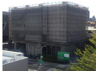
Station G8: Exits/ Entrances construction at Wenxin Rd. and Yinghua Rd. intersection
