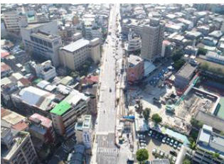
Stage 5 MOT area
