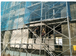
Station G09-1: insulated concrete panels installation on outer wall and painting
