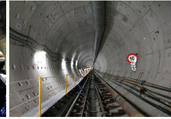
Station LG02-Station LG01 down track in shield tunnel
