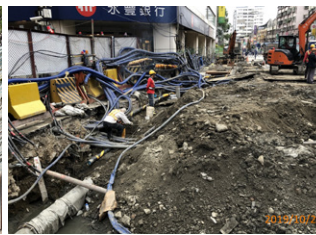
Pipeline moving at Central pocket tracks
