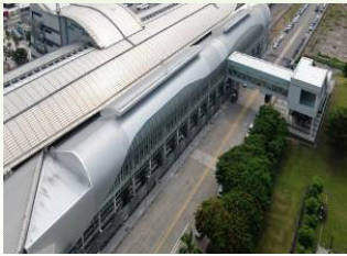
Construction status of Station G17 with entrances/exits along Jianguo Rd.
