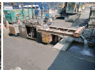
CP6 tunnel cross-passage Stage-3 traffic maintenance (diaphragm wall special unit work)
