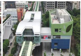
Current construction of Station G12 with entrances/exits along Wenxin Road
