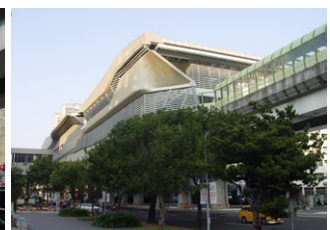
Construction of Station G9 from Taiwan Boulevard to Dalong Road
