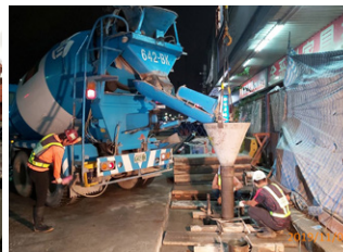
Concrete placing to form diaphragm wall of the cut-and-cover tunnel on Jincheng Rd. Sec. 3
