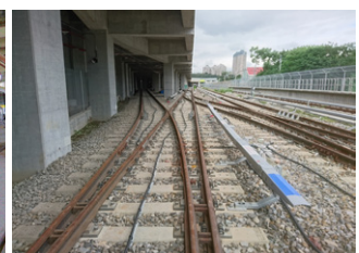
Completed track and conductor rails at South Depot
