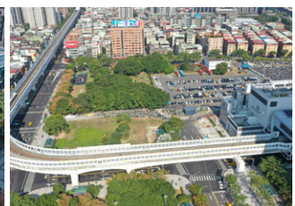
Elevated section of Banqiao Station (Circular line)
