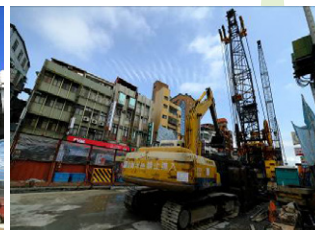
Diaphragm wall construction to the east of the central shelter line
