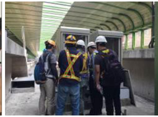
PWR, track-side equipment handover
