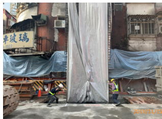
Station LG08 Rebar cage hoisting and placing for diaphragm wall
