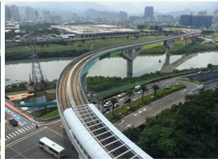
Cross-river steel bridge
