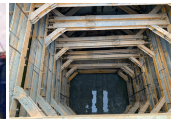
Retaining support and decking construction for the tail track working-well at Yucheng Park
