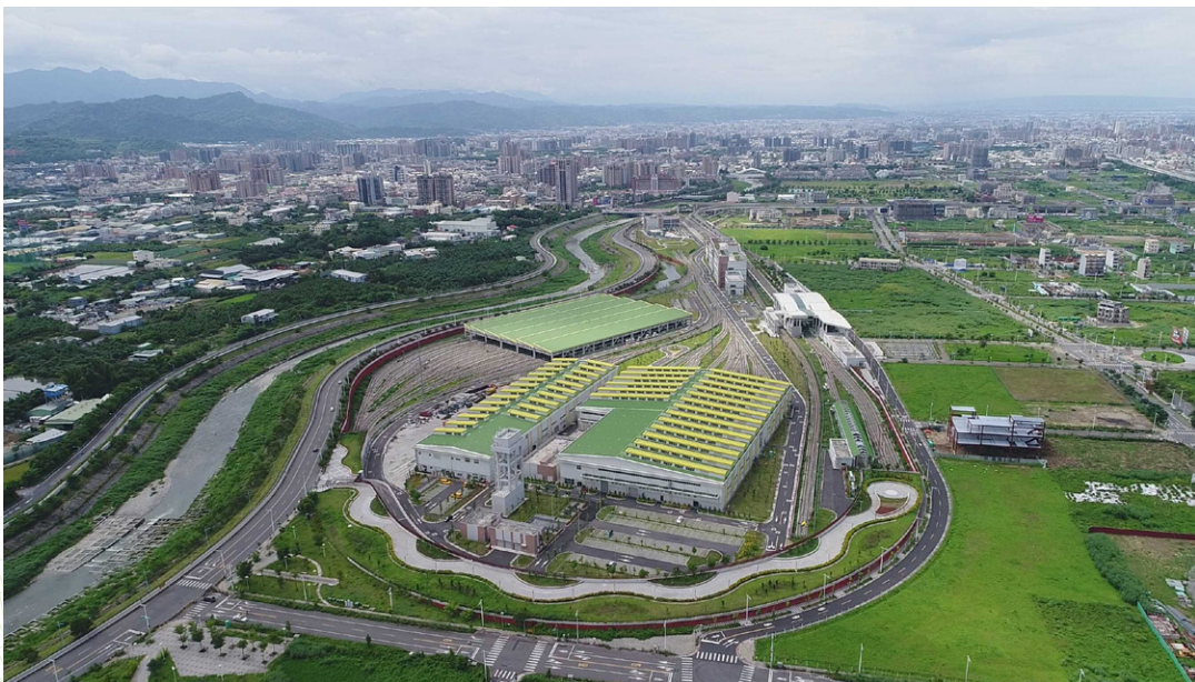
Aerial shot of the entire construction area
