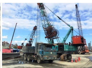
Diaphragm wall excavation at management center (Area 5)
