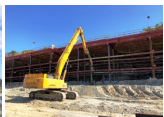
Steel pile work at Maintenance Area (Area 6)
