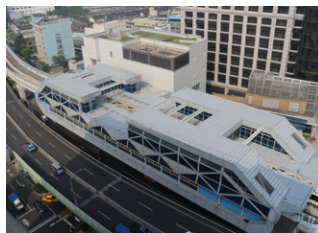
Bird's eye view of Touqianzhuang Station (Y17)
