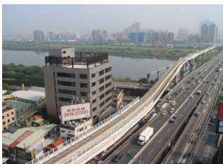
Touqianzhuang Station (Y17) southbound viaduct across the Dahan River Bridge Section
