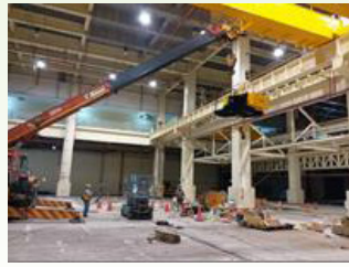
Hoisting the overhead crane at Xinzhuang Depot
