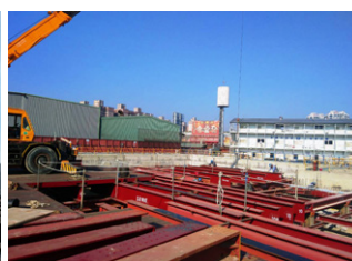
Supporting work at Station LG08A (Area 3)
