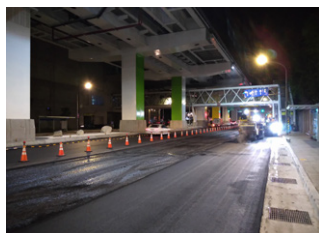
Asphalt concrete paving
