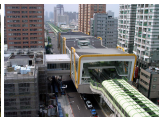
Construction of Station G5 from Chongde Road to Hebei Road
