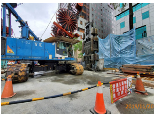
diaphragm wall digging work at Central pocket tracks
