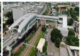
Construction status of Station G16 with entrances/exits along Jianguo Road
