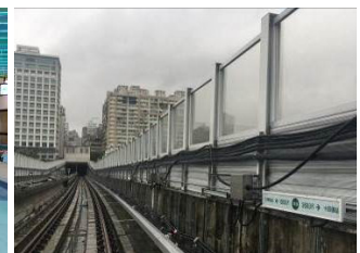
Sound barrier for daylight section
