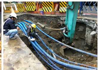
Pipeline moving for Station LG08
