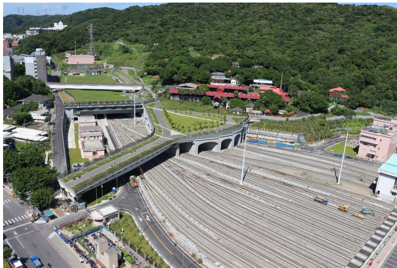
Bird's-eye view of the construction status of Xinzhuang Depot
