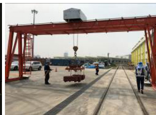
Depot equipment, gantry crane on-site test
