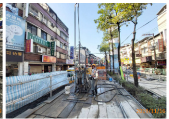
Stratum improvement for passage to Liancheng Rd
