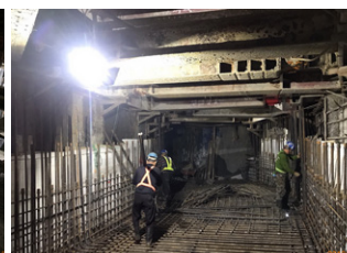
Rebar tying for the base plate of linking passage
