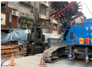
Station LG08 diaphragm wall digging work
