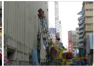
Station LG01 diaphragm wall work
