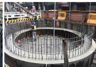
CP7 tunnel cross-passage Stage-2 traffic maintenance-- caisson work (concrete pouring after the assembly of cutting edge at the bottom)
