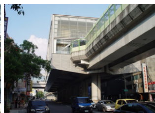
Construction of Station G8a from Yinghua Road to Xitun Road
