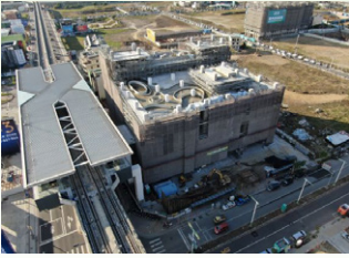
Aerial shot of Station G3
