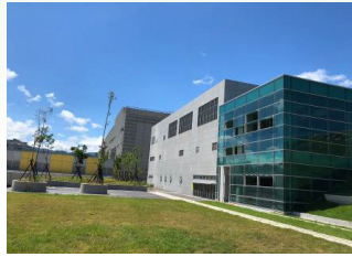
Shisizhang Station and landscaping platform
