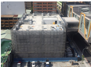
Station G5: Exits/ Entrances construction at Wenxin Rd. and Tianjin Rd. intersection
