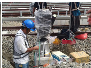
Xinzhuang Depot signal installation and connection
