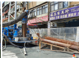
Construction of pilot hole for the diaphragm wall north of Station R03
