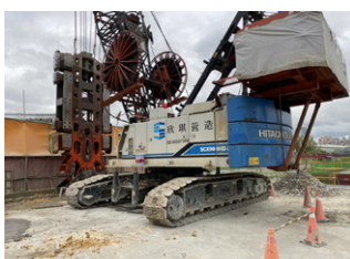
Diaphragm wall excavation at cut-and-cover tunnel (Area 4)
