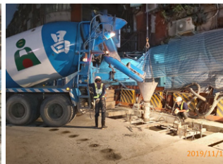
Concrete placing for diaphragm wall of station LG08
