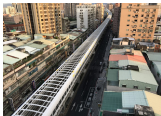
The Construction of sound barriers of the original contract at Banxin Rd.
