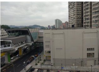
Xiulang Bridge Station and land development building
