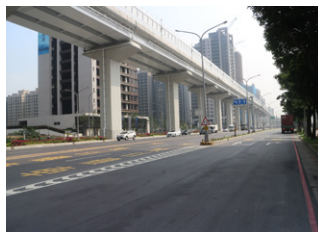
Elevated section between Xingfu Station (Y18) and New Taipei Industrial Park Station (Y19)
