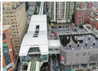
Current construction of Station G11 along Wenxin Road
