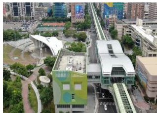
Current construction of Station G10 with entrances/exits along Wenxin Road
