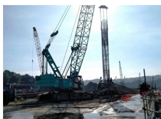
Pile and rebar cage connection on Stock yards (Area2)
