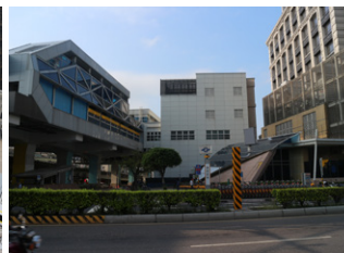
Connecting passage (O3) between Y17 and O3 Touqianzhuang Station (Y17)
