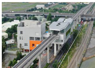
Construction status of Station G14 with entrances/exits along Jianguo Road
