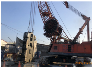
Diaphragm wall digging for cut-and-cover tunnel on Jincheng Rd. Sec. 3
