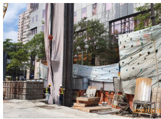
Rebar cage forming for diaphragm wall at Central pocket tracks
