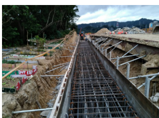
Retaining pile and tie beam work at east side of the road (Area 1)
