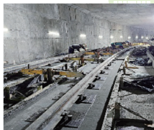
Ballastless bed concrete foundation work between Station LG08 and LG08A
