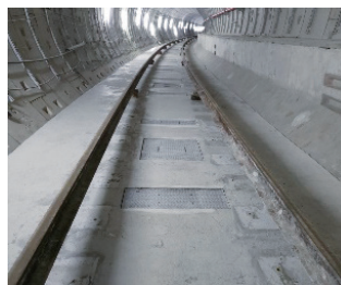
Floating slab completed between Station LG06 and LG07
