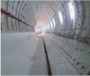
Up/down track tunnel completed for LG07-LG06
