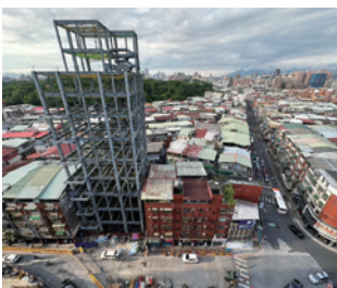
Steel structure erection completed for Station LG08 Exit A
