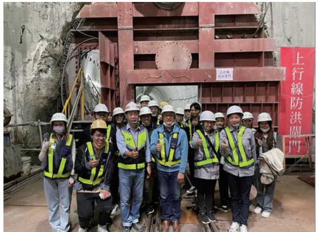
Photo 14: National Central University visited contract CQ850 construction site (November 13)
