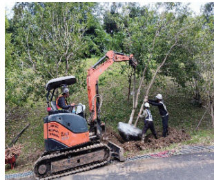
Station Y1A tree displacement work at Zhuangjing Residence, NCCU
