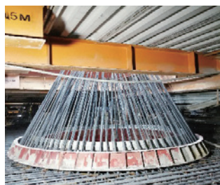
Station shaft for light and ventilation
