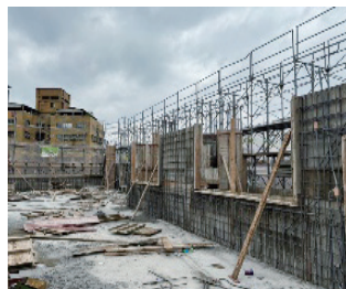
Social Welfare Building 6F structure work
