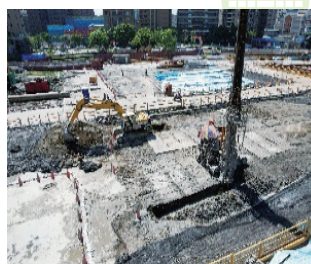
North Depot foundation improvement work
