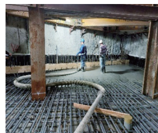
CP6 vent shaft B1 plate concrete placing work
