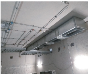
Wind pipe and electrical conduit work at low-voltage substation, Station LG06
