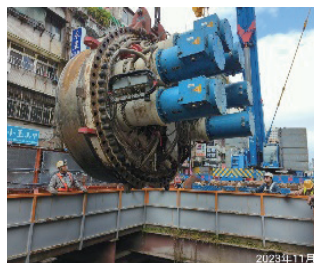
Installation of the driver to shield machine
