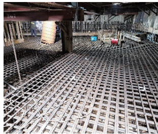
Rebar tying work of the concourse plate at Station LG01
