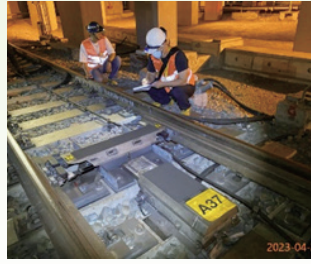
Night inspection of South Depot track area equipment
