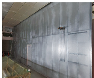
Soundproof work for server room at equipment level, Station LG02
