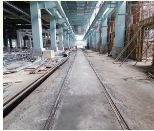
Maintenance yard track work
