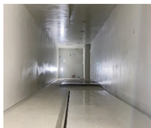
Painting work for partition wall at Station LG05
