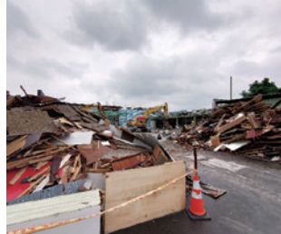
Removal of existing buildings
