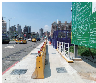
Station Y22 sidewalk narrowing
