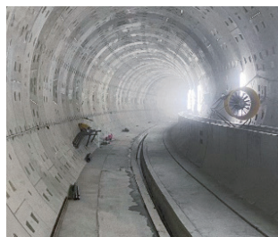
Down track tunnel completed for Station LG08 cut-and-cover section
