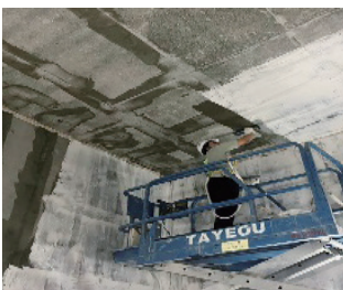
Ceiling mud work in the non-public zone at LG03
