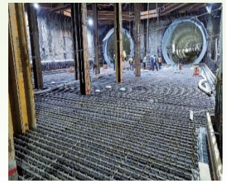
Station R01: structure work
