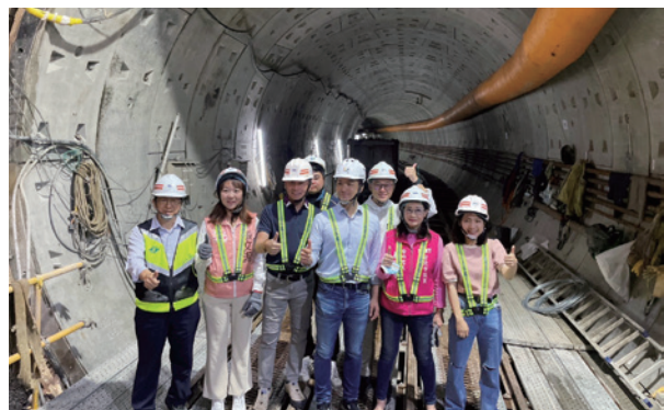
Photo 6: Mayor Chiang Wan-an inspected the construction progress on Xinyi eastern extension (April 10)
