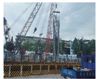
Station Y23 steel cage placement for diaphragm wall
