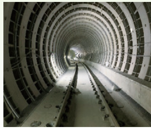
R01 west shaft down track: track laying
