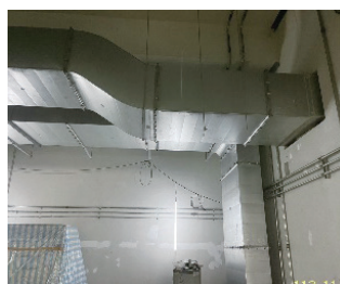
Server room pipe work handover
