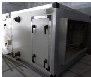
AHU arrival at the equipment level
