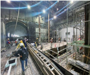
Structure work for the south shaft
