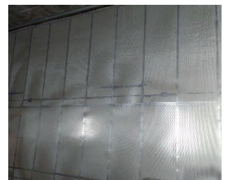
Soundproof work in the server room
