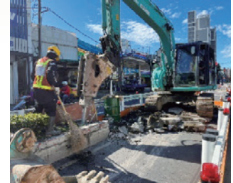
Removal of median refuge island from Zhonghua Rd.
