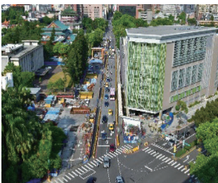
Birds-eye view of the CQ842 construction site
