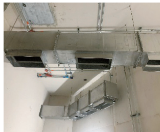
Wind pipe and electrical conduit work at battery room, Station LG06
