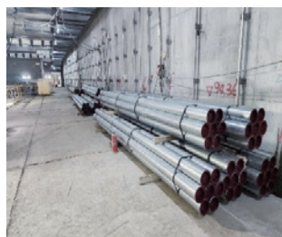
Galvanized steel pipes arrived at Station LG03
