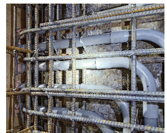
B1F grounding pipe embedding, Station LG08 Exit A
