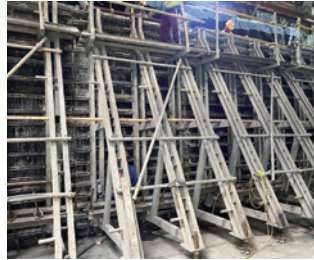
Structure formwork adjustment for Station LG07 sidewall
