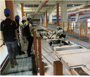
Circular line Phase I EMU compatibility inspection
