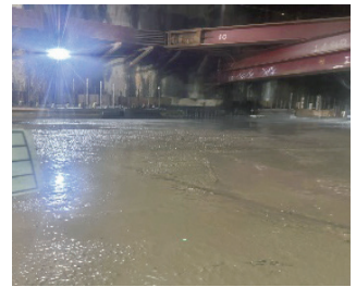
Concrete placing of the concourse plate at Station LG01
