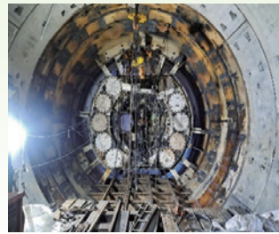
R01 east shaft downtrack: shield machine disassembling
