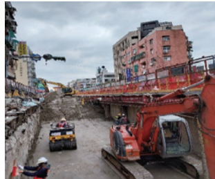
Station restoration work
