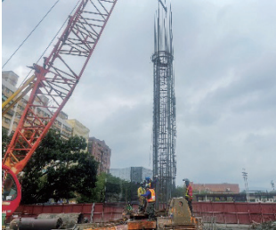
Station LG14 foundation pile work
