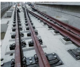
Installation of switch track floating slab between Station LG08 and LG08A
