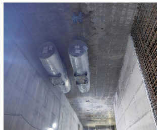
Installation of jet fans
