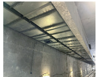
Exhaust pipe and OTE wind pipe installation, upper platform, Station LG06
