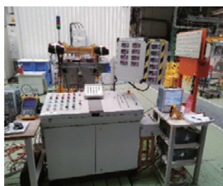
EMU static inverter testing
