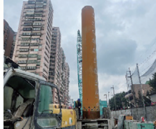
Daan Rd. foundation pile work
