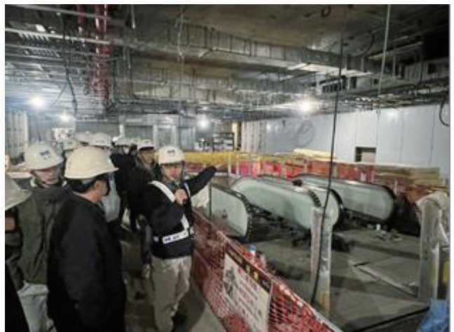
Photo 16: Chung Hua University visited contract CQ870 construction site (December 22)
