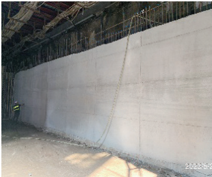
Sidewall completed at B1 concourse level of Station LG06
