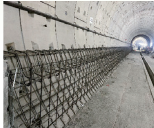
Walking path work inside tunnel
