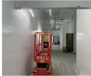
Decoration work inside Station LG07
