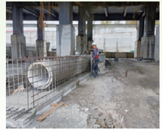
Drainage work for the ground of the roundhouse
