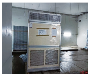
Placement of AHU at the platform level
