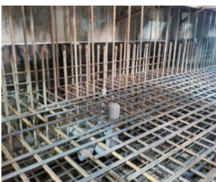
Drainage work at the concourse level of Station LG01
