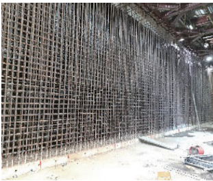
Rebar tying work of the concourse side walls at Station LG01
