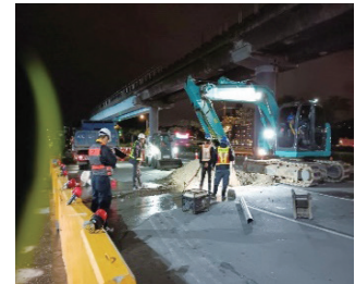
Station Y1 pipeline trial excavation
