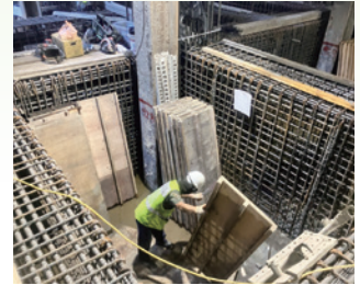
Underground structure work, Station LG07 Exit B
