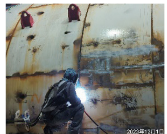
Welding work of the shield machine shell
