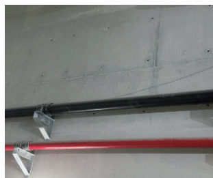
Fire extinguishing pipe and drainage pipe work, Station LG07 - LG08 tunnel
