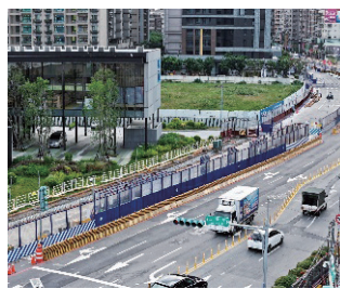
Station Y22 fence set up for traffic routing
