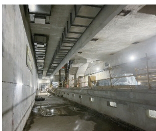
Platform exhaust pipe installation
