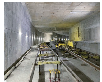
Up/down track tunnels completed at the cut-and-cover branch
