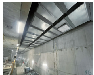
Installation of ventilation pipes, platform level, Station LG03
