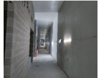
Partition wall work inside station
