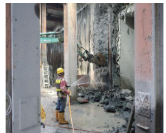
Exit B-B2F diaphragm wall opening removal work
