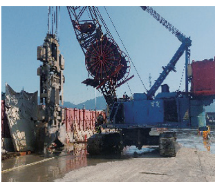
North Depot diaphragm wall work
