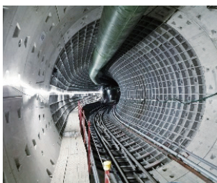
Shield tunnel advancing along the down track
