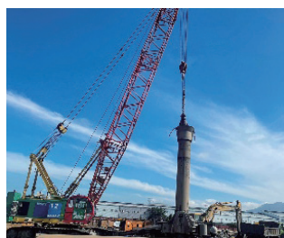
North Depot center post work
