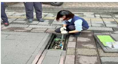
▲ Flood Control Operations
