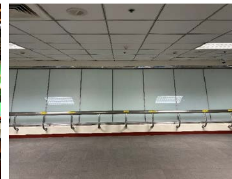
▲ Addition of New Electronic Privacy Film in the Operations Control Center Observation Area
