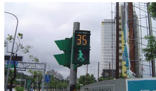
Little Green Men - Countdown Pedestrian Signals.
