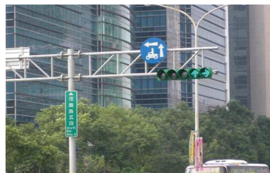
Upgrading traffic signals with LED lights and aluminum light cases.
