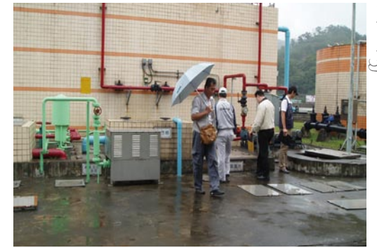
Inspecting a sewage treatment facility.
