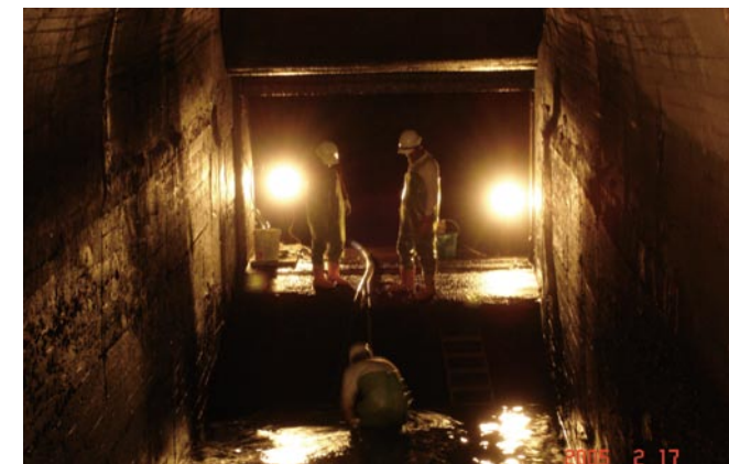
Inspection work of the Qingtan Weir Unfiltered Water Transmission Mains.
