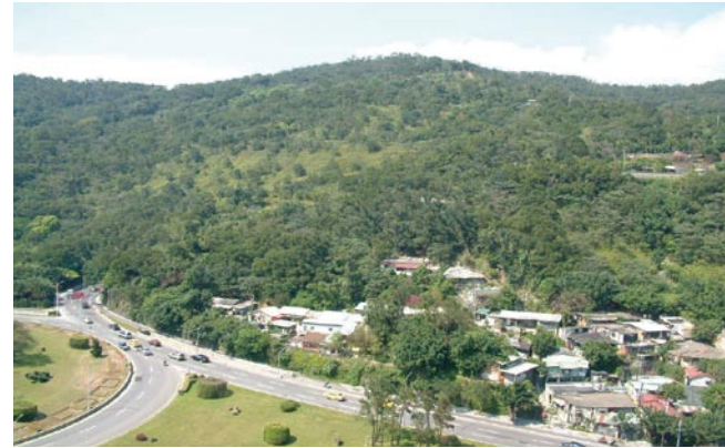
At the Foot of Jinan Mountain located on the east side of the Ziqiang Tunnel’s South Exit, before the village was demolished.
