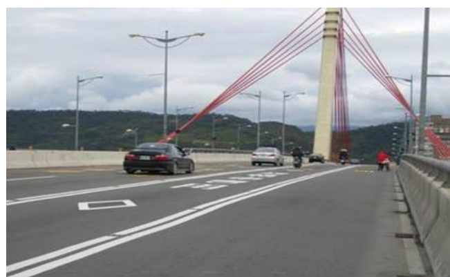
Motorcycle and slow-moving vehicle lanes on Dazhi Bridge (heading toward Dazhi).
