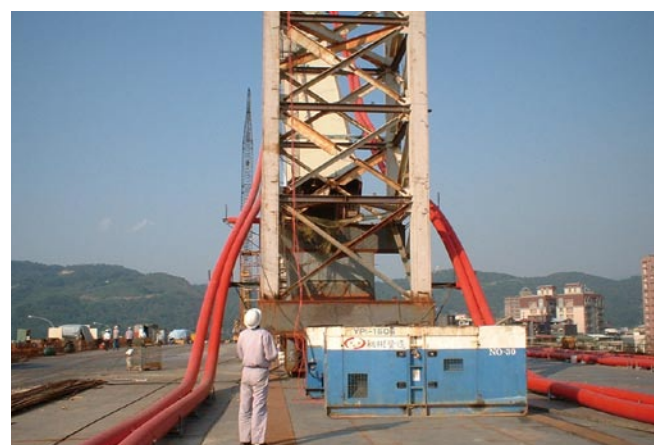
Inspection of Dazhi Bridge.
