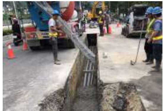
Incinerating recycled aggregate for road excavation
