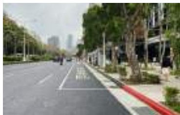
Porous asphalt concrete pavers along Zhongxiao E. Rd.
