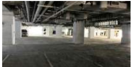
Illegal building after improvement
