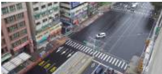
Roosevelt Road bus lane (after construction)
