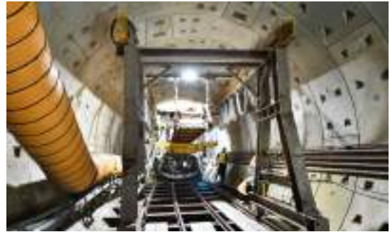
Tunnelling shield at the Xinyi Line eastern extension
