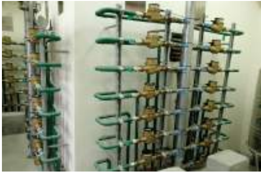
Smart water meter installation and testing
