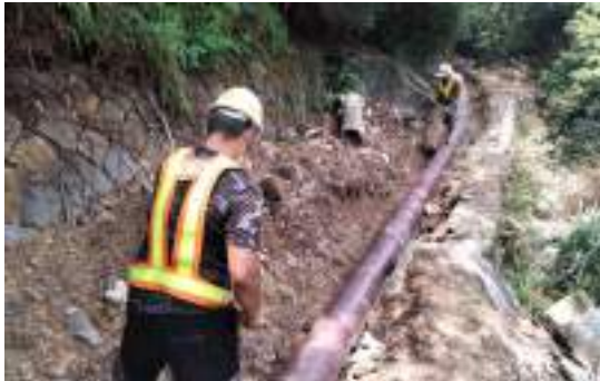
Maintenance and replacement of the hot spring pipelines
