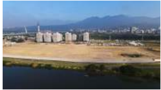
Grading and leveling works in Phase 2 of the Beitou-Shilin Technology Park completed
