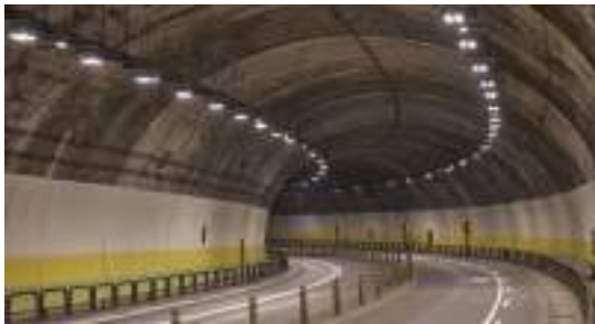
Replacement with LED lights in Kangle Tunnel
