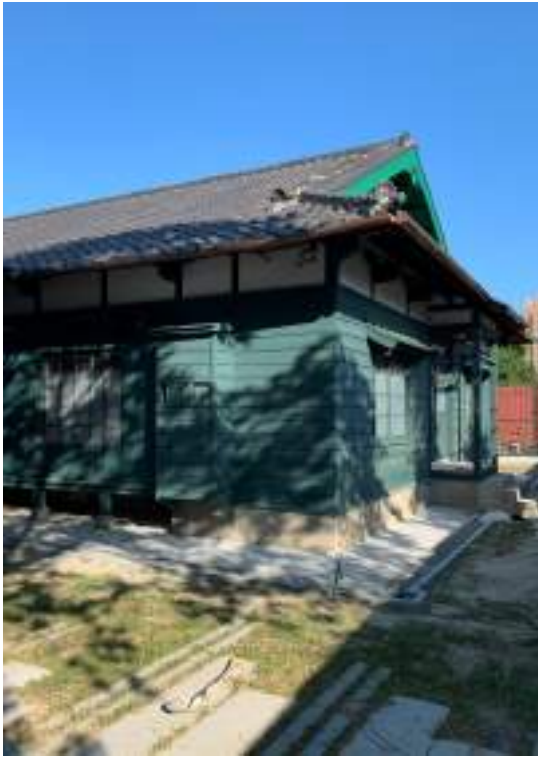
Jiahe New Village Restoration
