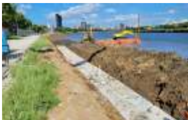
Reuse of local materials such as stones
