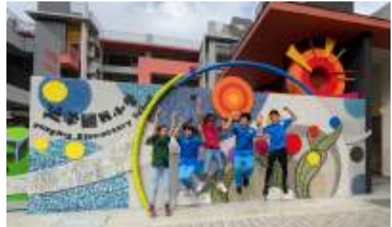
School buildings combining aesthetics, ecology and energy saving
