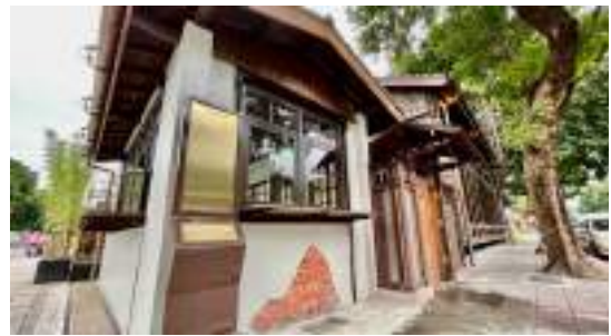
Former Taipei Prison dormitory (3 Aiguo East Road)
