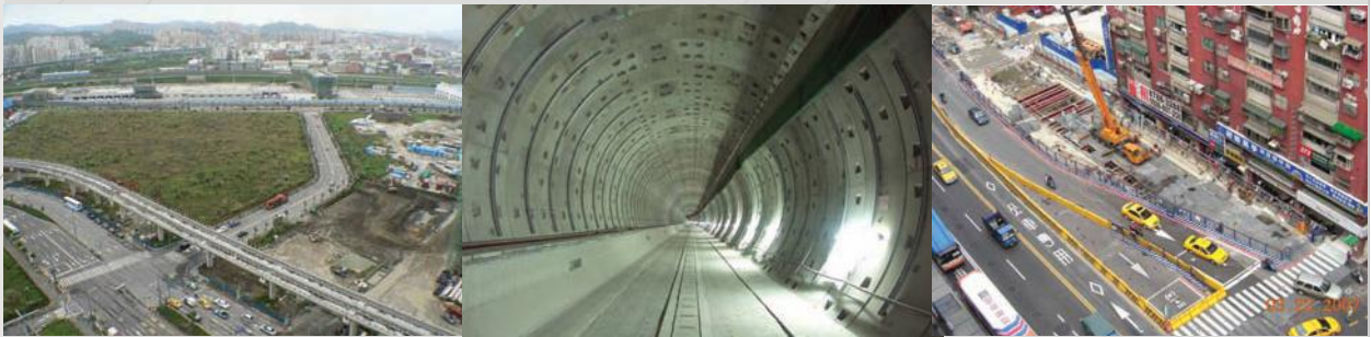
• Birds-eye view of Neihsu maintenance depot from the Neihsu line
