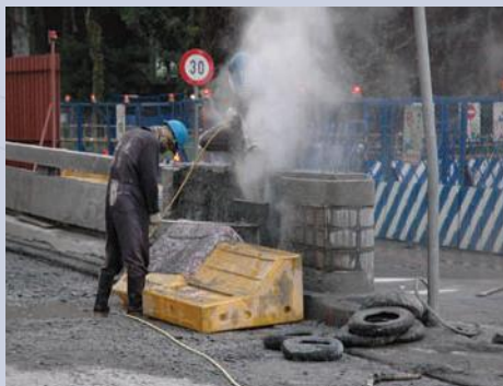
● The demolition of Guanghua Bridge
