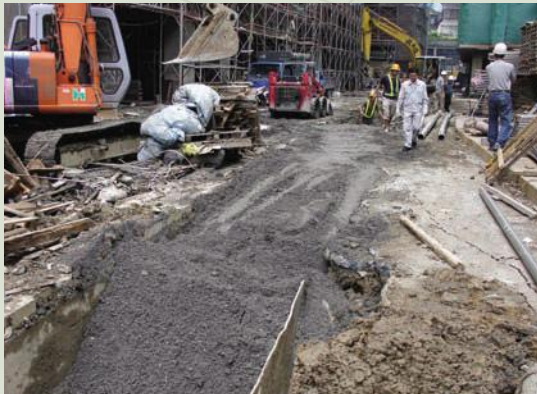
● Bottom Ashes Reused and processed — telecommunications pipes backfilled
