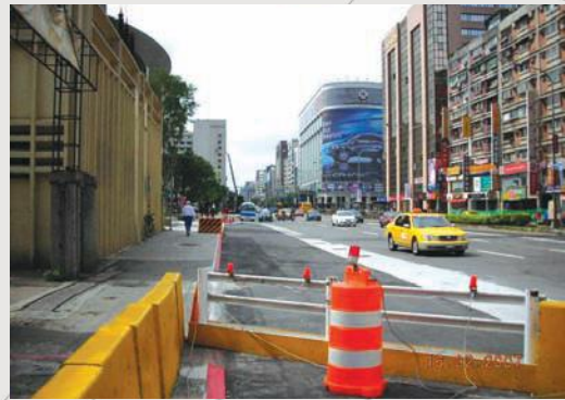
● Footpath narrowing work on Songshan line
