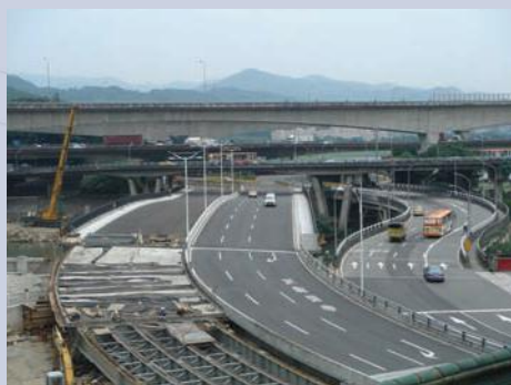
● The New Zhongshan Bridge under construction
