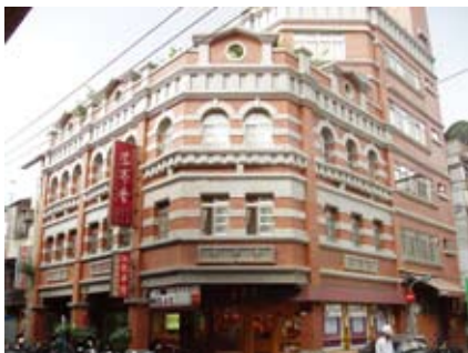
Post Improvement Condition of Lee's Cake Shop.
