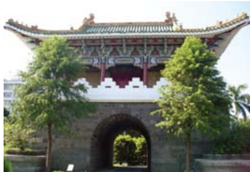
Taipei's South Gate following renovations.
