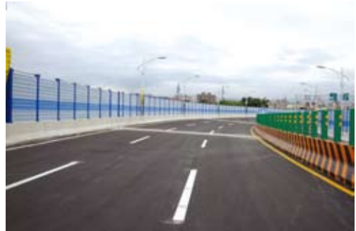
A smooth, driver-friendly Xinsheng Viaduct.
