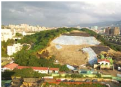
Panoramic view of the construction site where the Neihu Garbage Mountain was removed.
