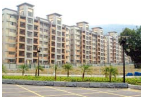
Expropriated housing for the designated Shilin Presidential Project.
