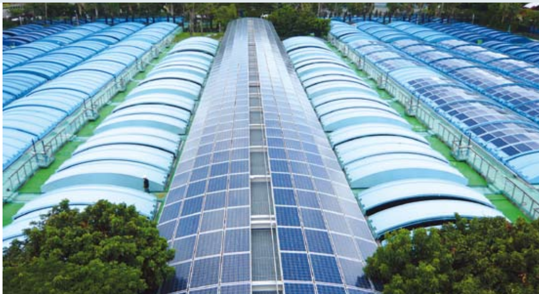
Photovoltaic Power Generation System in the Gongguan Purification Plant.
