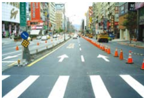
Level surfaces of city roads..
