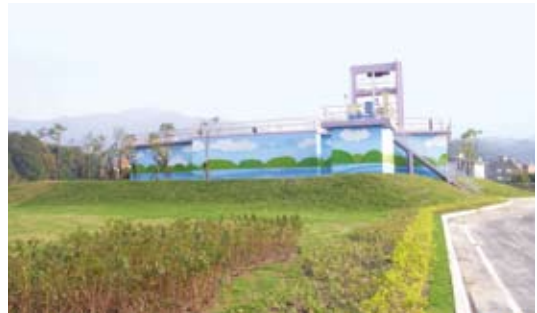
Gravel-removing spillway well of the 2nd Untreated Water Transmission System Project.
