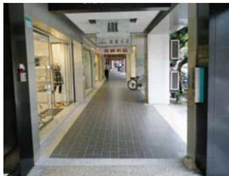
Post-improvement of Bei-An Road Walkway.
