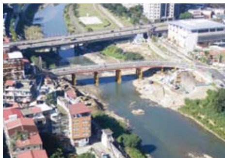
Jingmei Bridge under construction.
