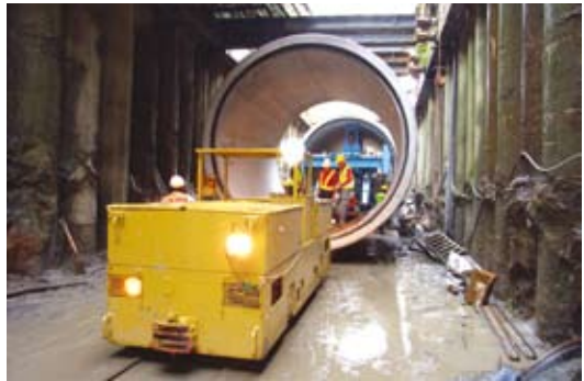
The 2nd Untreated Water Transmission System Project pipe jacking work for the tunnel.
