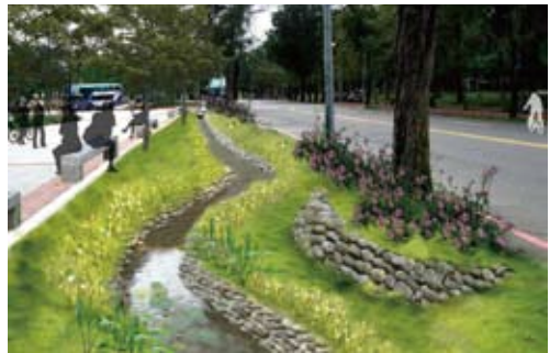
Post Improvement of the Ditch at Shilin Chiang Kai-shek Official Residence.
