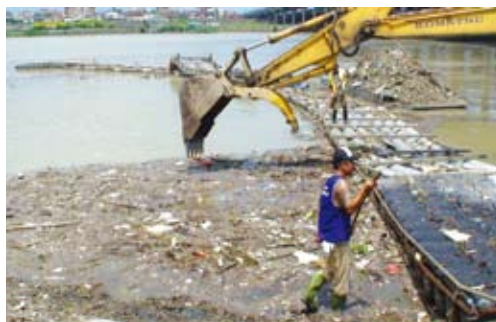
Garbage on the river surface was removed, followed by a cleaning treatment
