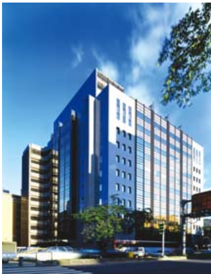
Post Improvement Condition of Guangfu Building.
