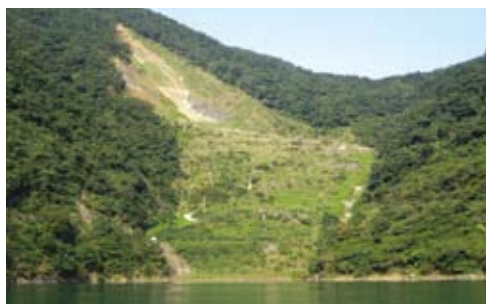
Collapsed locale in the Feitsui Reservoir's catchment area is successfully renovated.
