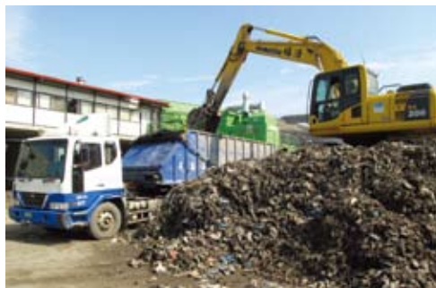
The removal of the Neihu Garbage Mountain – on-site.
