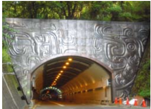
Wall surface beautification (eastside) inside Tzechiang Tunnel.
