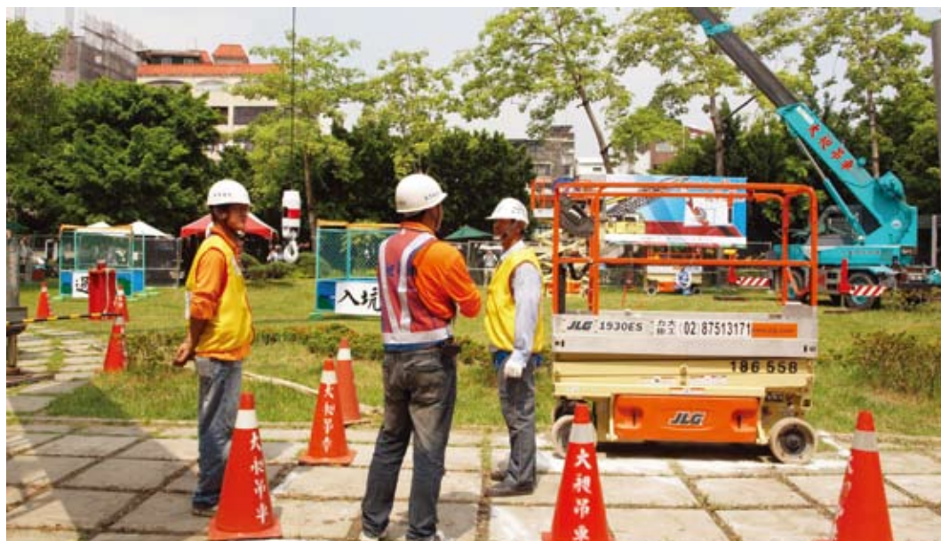
Crane operation technique competition and demonstration.
