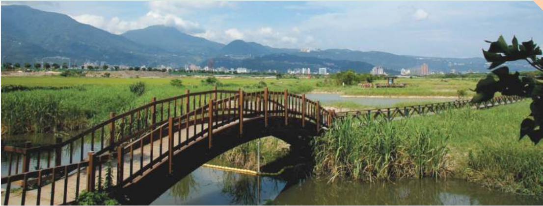
Constructed wetland by Shuimokeng Stream in the Guandu Nature Park
