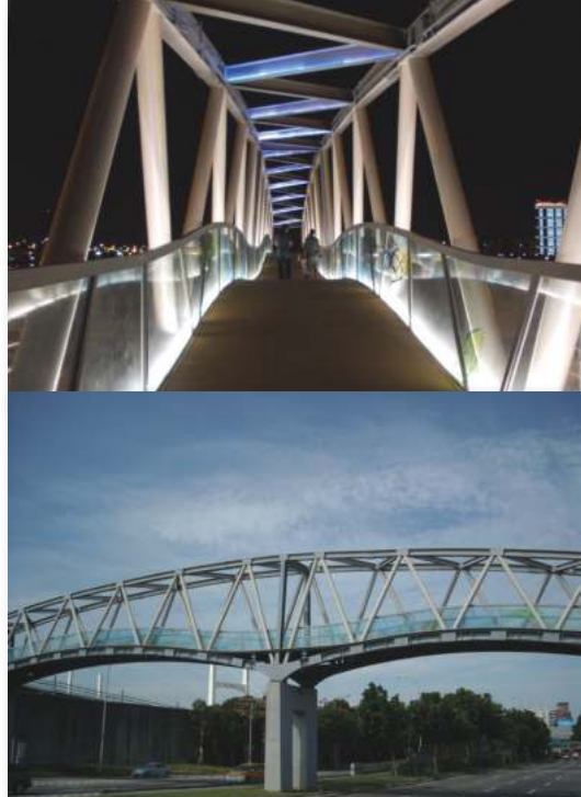
The pedestrian flyover by Hulu Elementary School
