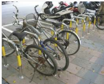
Γ-shape bar bicycle stand (suited for relatively narrow pavements)
