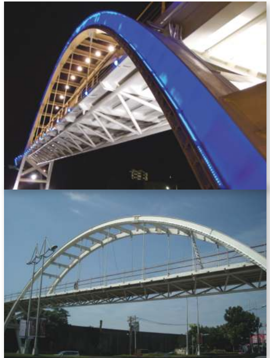
The pedestrian flyover by Shezi Elementary School
