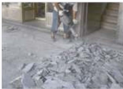
Stone-breaking (lead time: 1 day)
