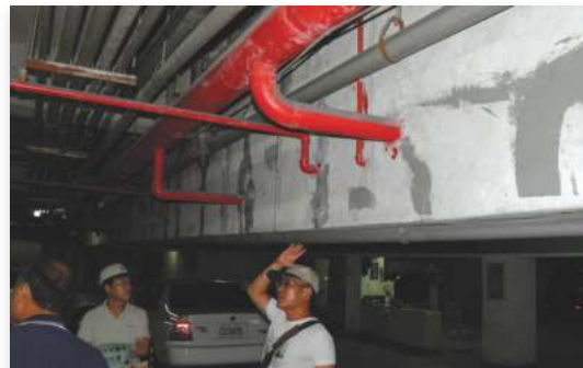
Uneven illumination due to deep beams in basement
