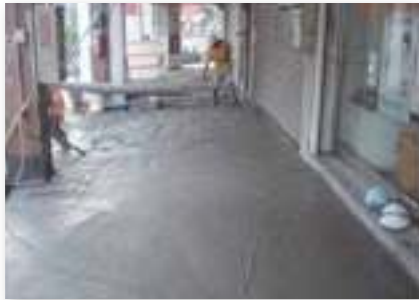
Cement-sand installation (lead time: 1 day)
