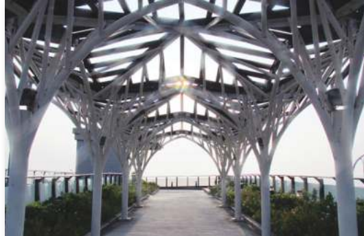
The entrance design at the park atop of Neihsu Wastewater Treatment Plant – the umbrage as guest reception
