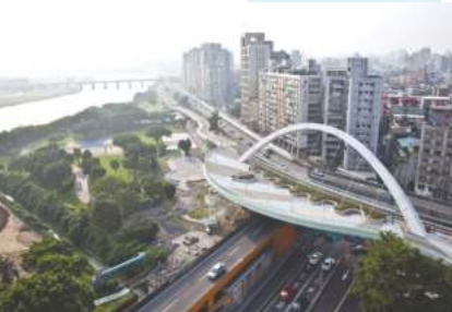
The construction of the Cross-Riverbank Pavement and Bikeway
