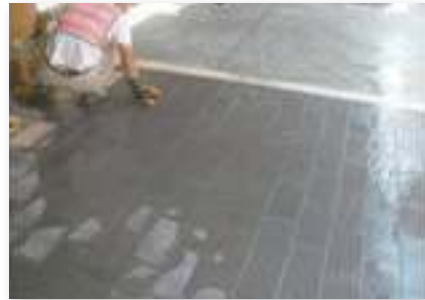
Tile grouting (lead time: 0.5 day)
