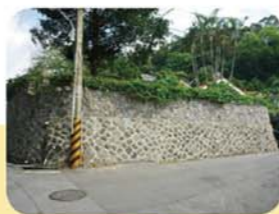
▲漿砌石擋土牆
