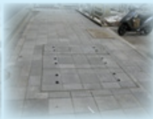
Sidewalk manholes along Nanjing East and West roads
