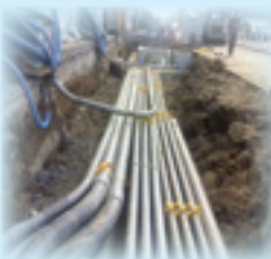
New pipelines beneath Nanjing East and West roads
