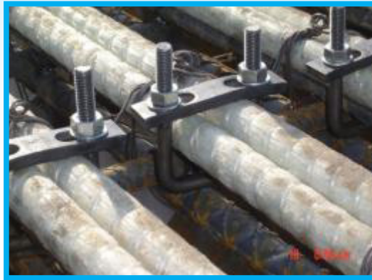
Glass Fiber Reinforced Plastic (GFRP) put in place
