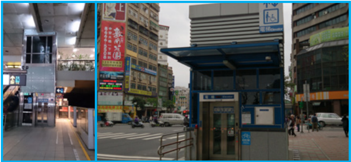
An elevator between the concourse and platform levels
