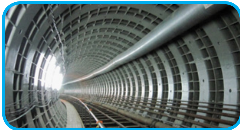
Completed spheroidal graphite iron rings in the shield tunnel
