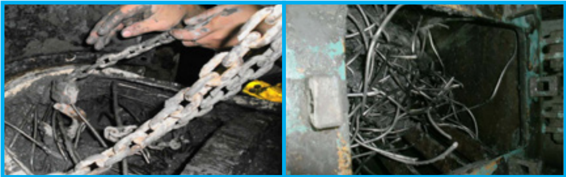
Anchor blocking at the inspection mouth after 1,000 mm of pulling by the shield tunneling machine screw axes
