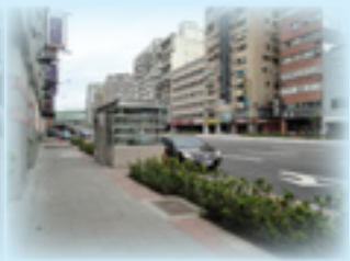
Rehabilitated sidewalk along Nanjing East and West roads
