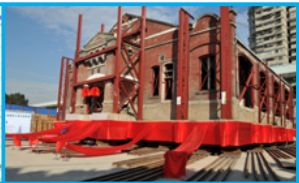
Taipei Workshop before removal
