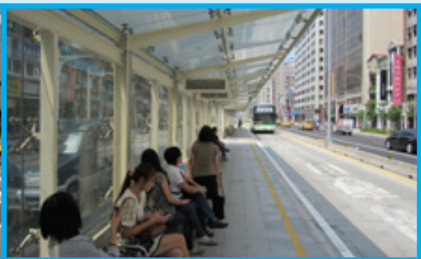
Compared to bus shelters along Xinyi Road, bus shelter glass roofs along Nanjing East and West roads better block the sun
