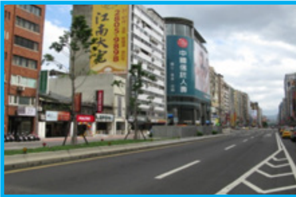
Median strips and common duct facilities
