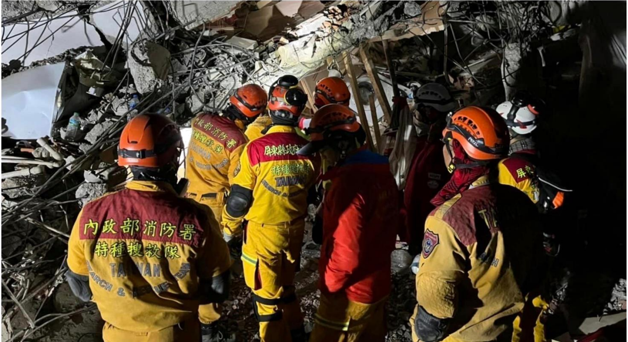
Schematic Diagram of Emergency Response for Disasters/ Source: National Fire Agency, Ministry of the Interior
