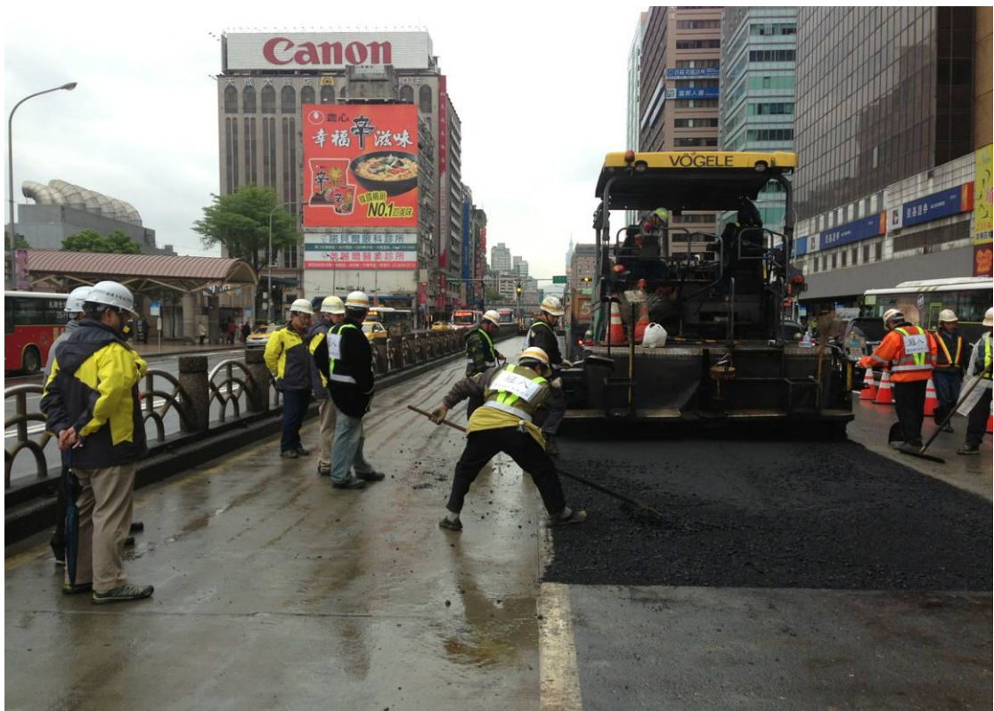
鋪裝機鋪設瀝青
