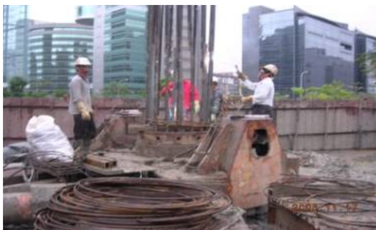
CB423標BSS(主變電站)鋼筋籠搭接
