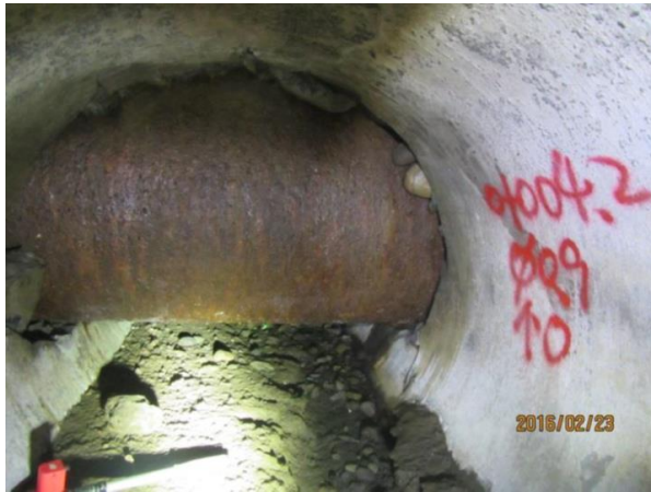
Fig.1 \phi 900mm water main penetrate pipe drain
