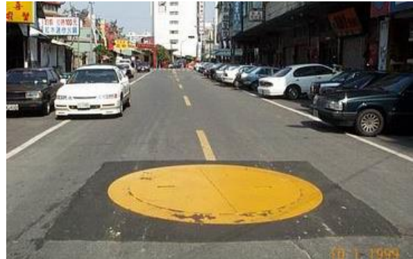
Fig.6 \phi 2.1M arrival shaft covered by plate
