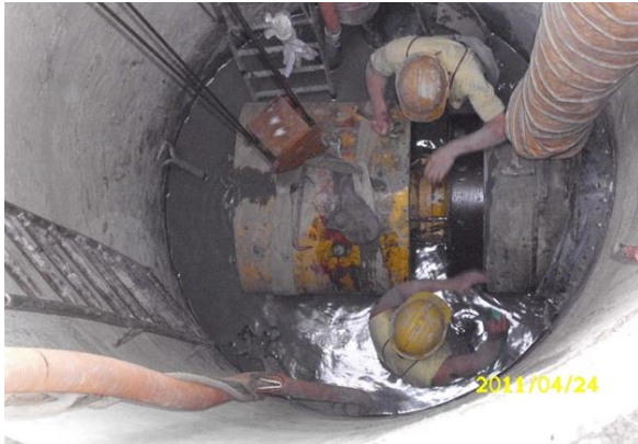
Fig.21 boring auger breakthrough arrival shaft
