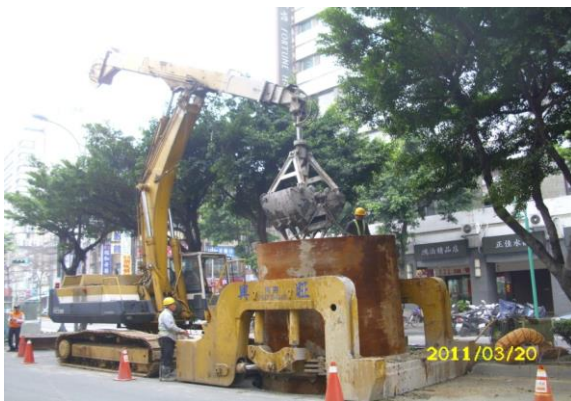
Fig. 19 excavation for steel shaft sinking
