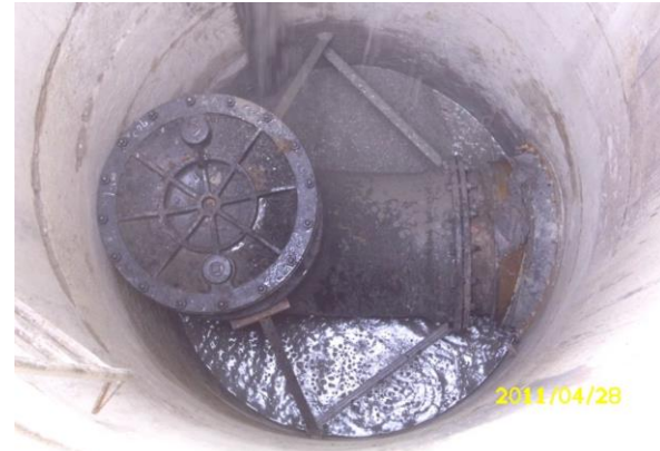
Fig.22 pipes fitting installed before pressure test
