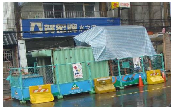
Fig.7 construction site of sewer jacking
