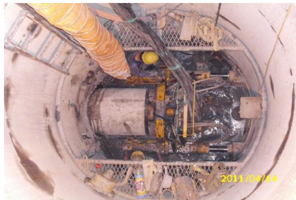
Fig. 20 circular steel-pipe made shaft
