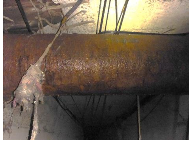
Fig.2 \phi 700mm water main penetrate box culvert
