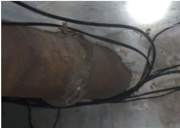
Fig.12 \phi 500mm DIP water main inside drain
