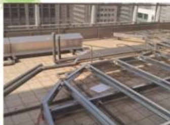
焊接C型鋼以架高木平臺
