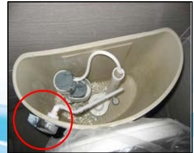
沖水桿卡住水箱水直瀉而流
