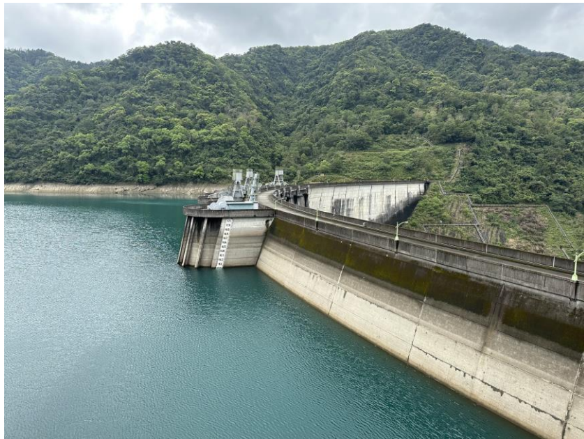
翡翠水庫預降水位，預留庫容，蓄洪防災
