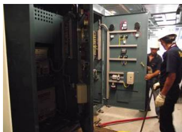
變頻器及配電盤安裝
